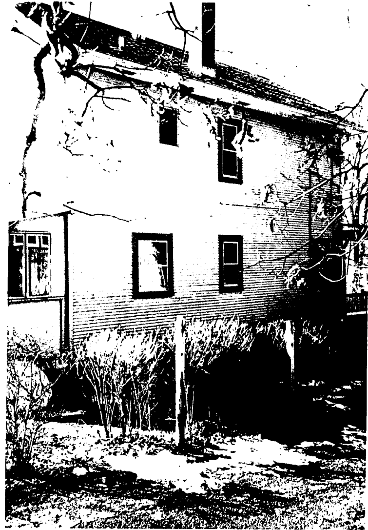
SIDE VIEW OF PROPERTY FROM NORTH SIDE OF THE LAWYER
