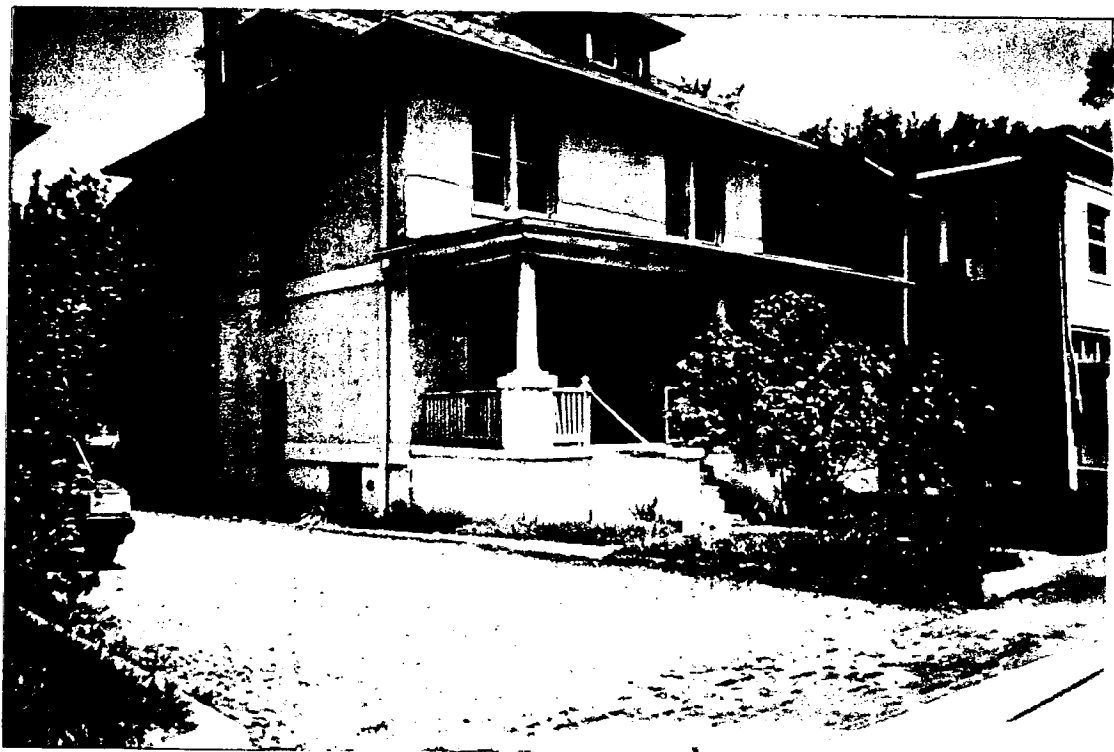
Adjacent Structure 7034 Carroll, Toward North-East
