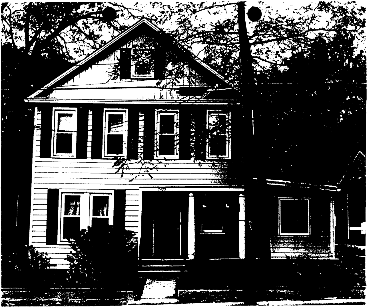
EXISTING HAUKESSIAN RESIDENCE -FRONT- ± 1:5
