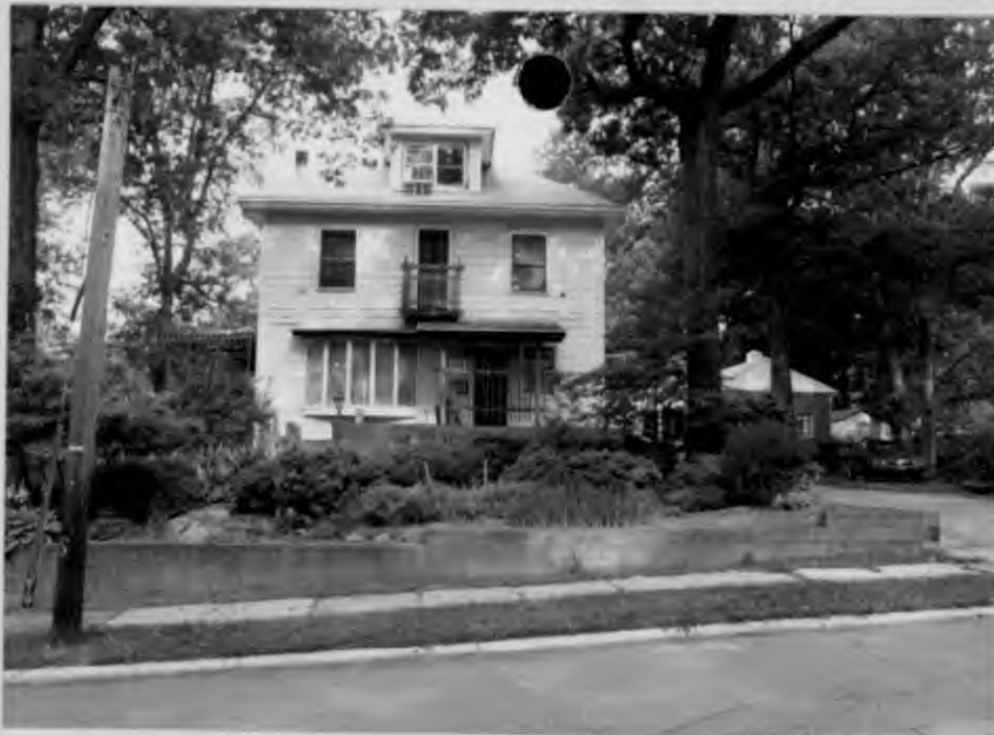
7416 Baltimore Avenue Looking west.
