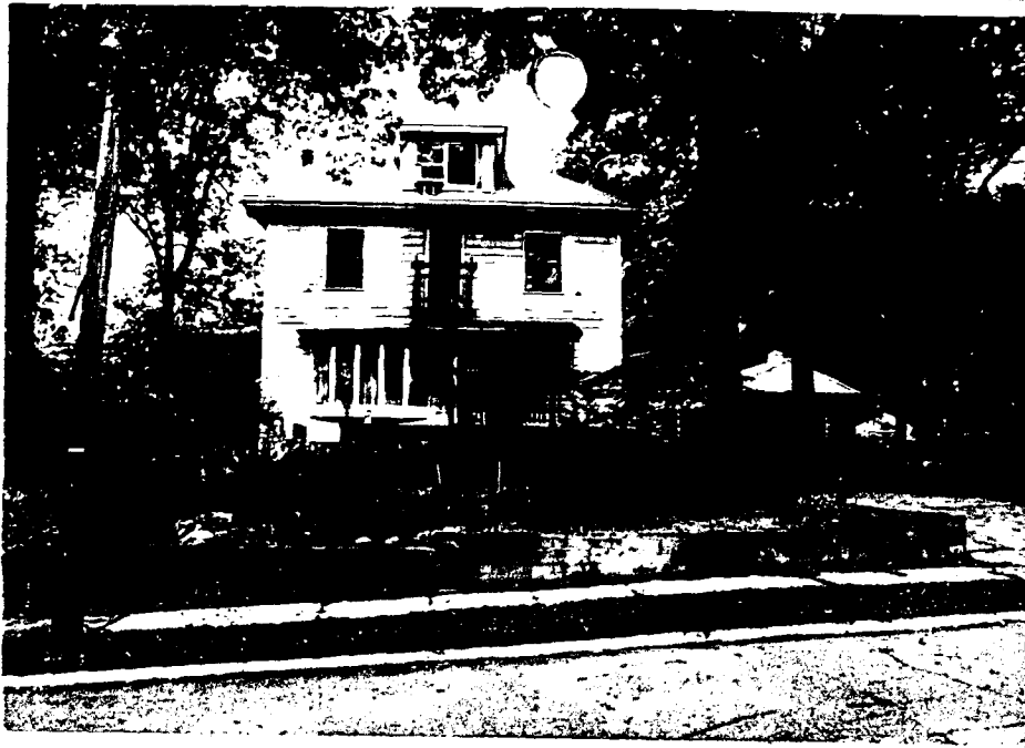
7416 Baltimore Avenue Looking west.
