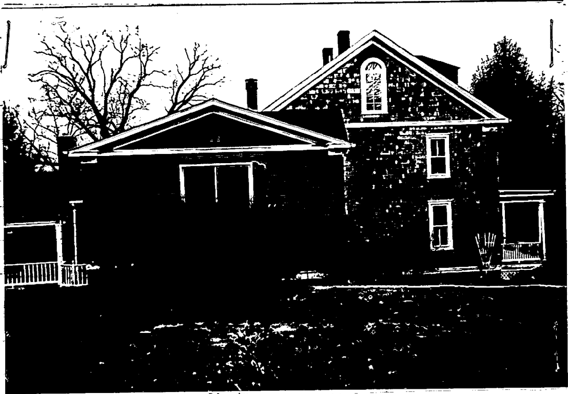
VIEW OF ADDITION AND HOUSE FROM WEST
