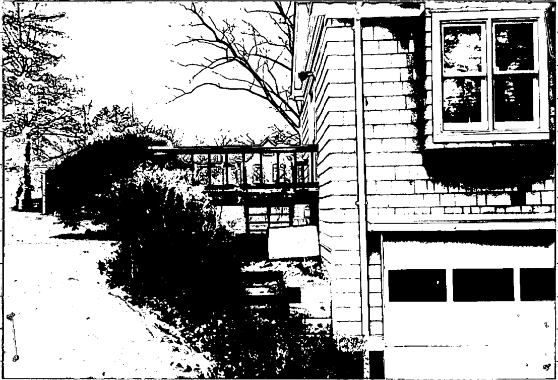
VIEW OF DECK FROM PROSPECT STREET
