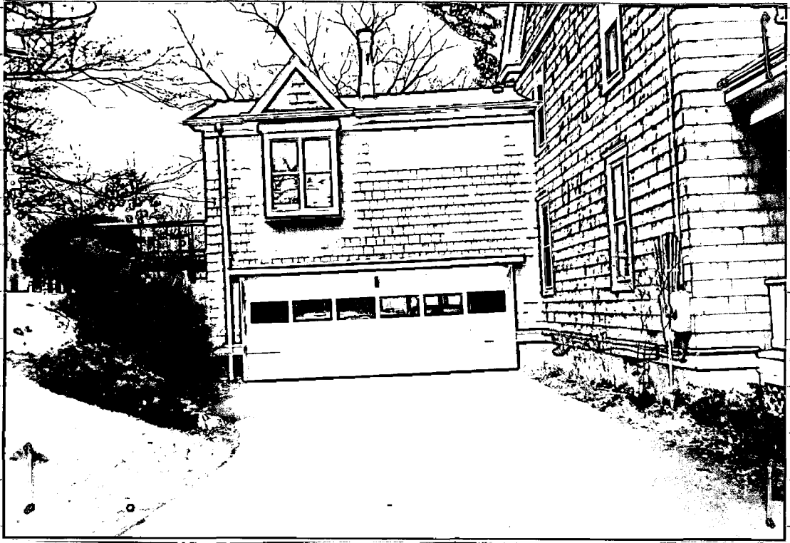
VIEW OF ADDITION (GARAGE/ MASTER BEDROOM) FROM PROSPECT STREET
