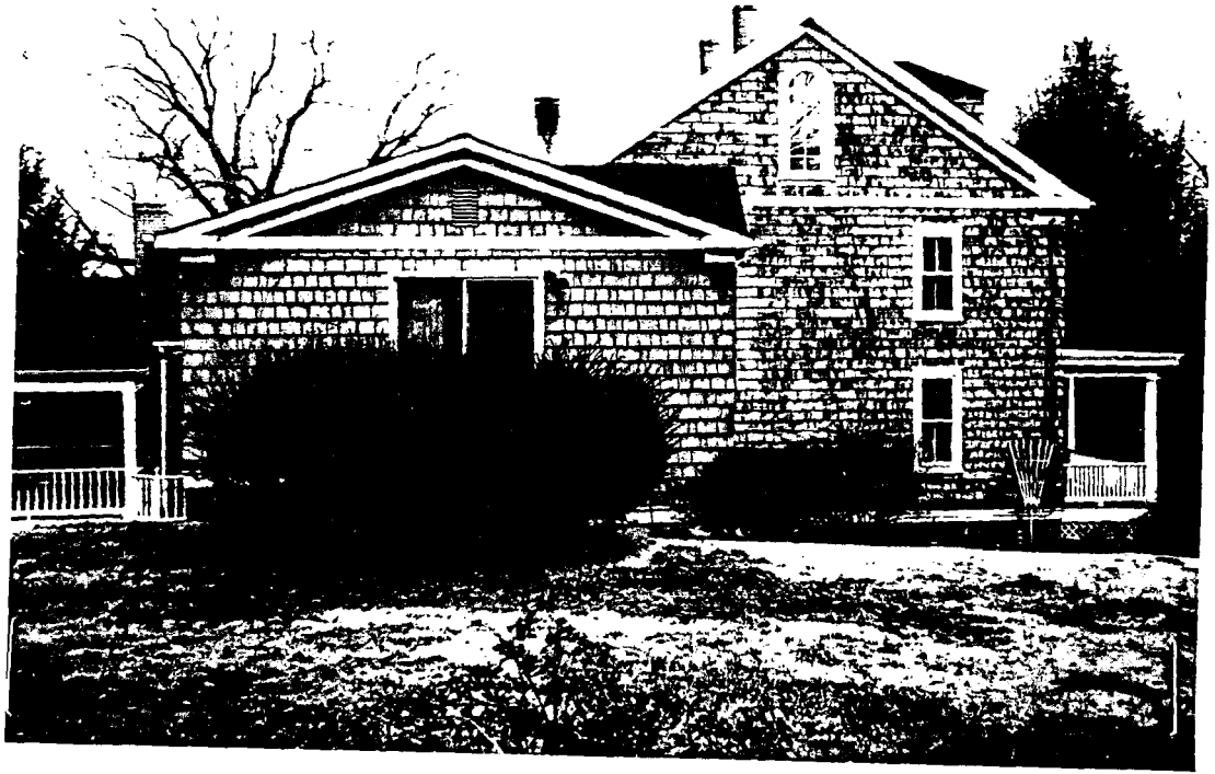
VIEW OF ADDITION AND HOUSE FROM WEST
