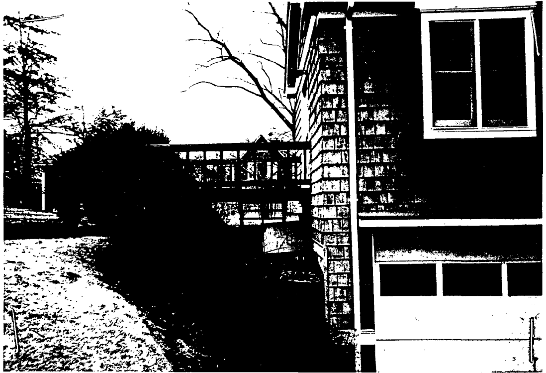
VIEW OF DECK FROM PROSPECT STREET
