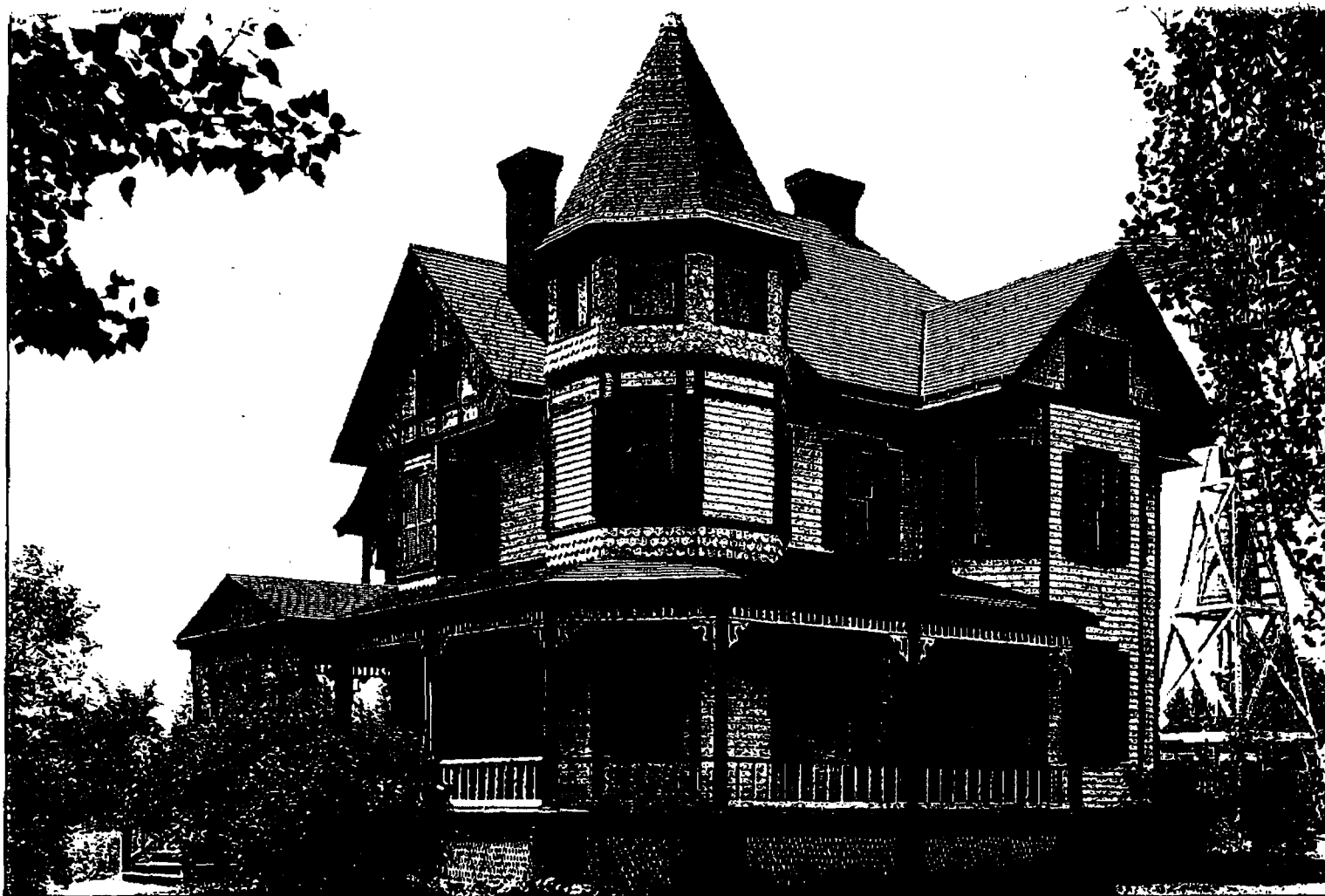
As with so many houses of its period, the trimwork on this Queen Anne Style house was painted in a contrasting color. The darker trim is now white, but the rich variety in wall texture is still apparent. Note the corner boards, decorative half-timbering on the front gable, use of both horizontal and vertical boards on the polygonal turret, and the spindlework ornamentation on the porch.
