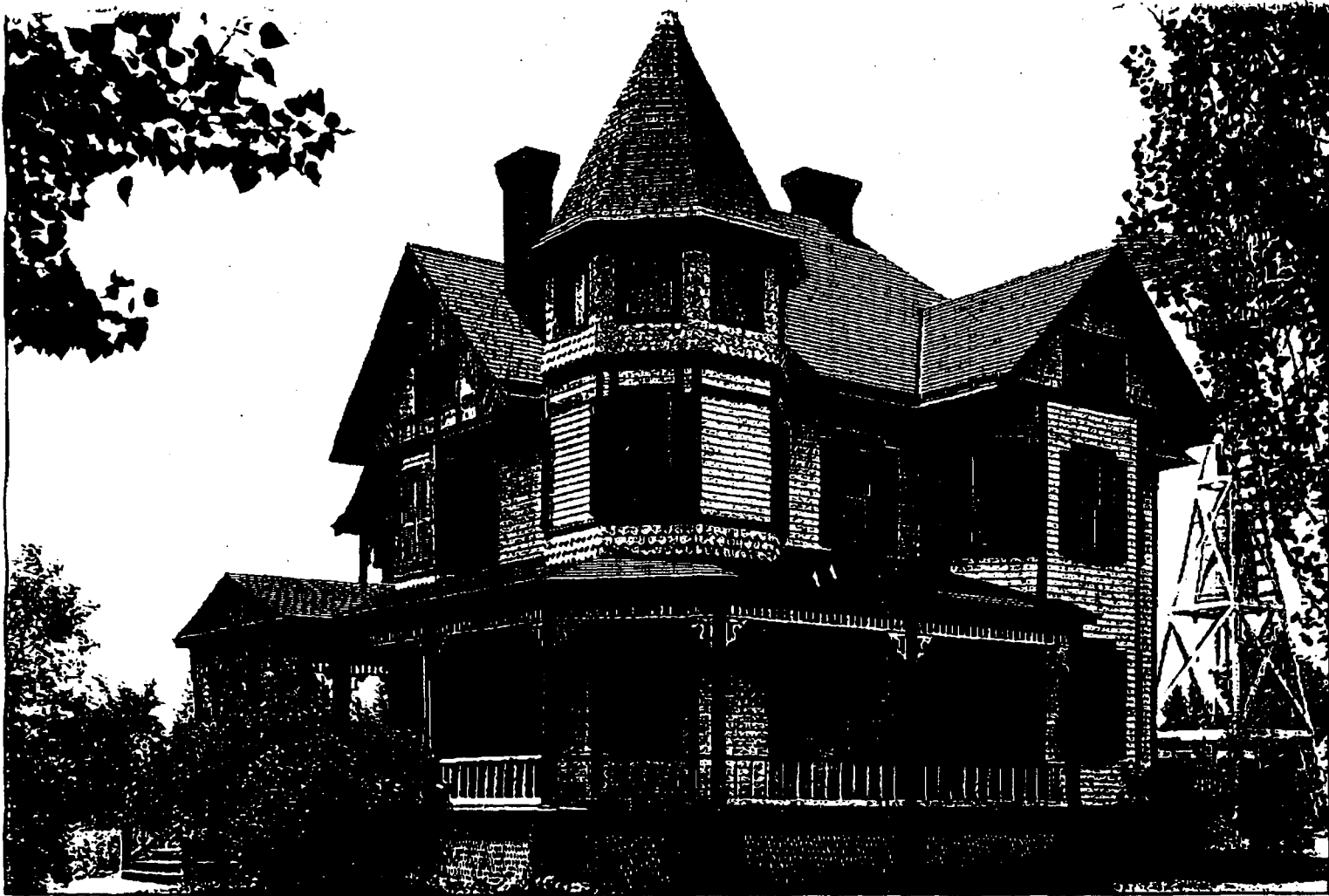
As with so many houses of its period, the trimwork on this Queen Anne Style house was painted in a contrasting color. The darker trim is now white, but the rich variety in wall texture is still apparent. Note the corner boards, decorative half-timbering on the front gable, use of both horizontal and vertical boards on the polygonal turret, and the spindlework ornamentation on the porch.
