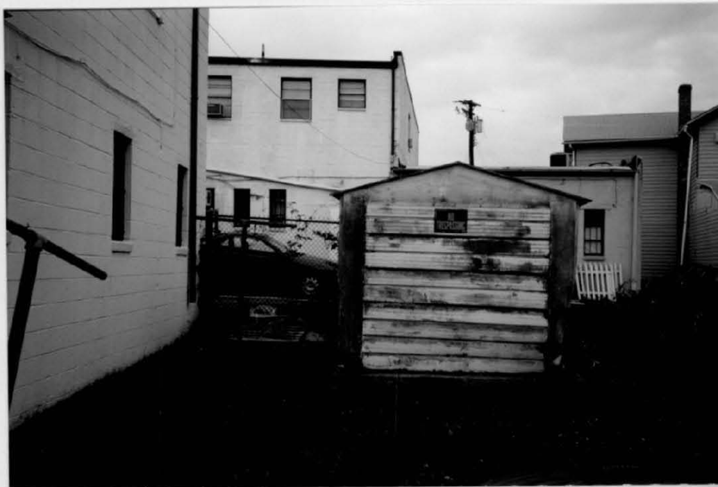
Existing shed as seen by Donohoe
