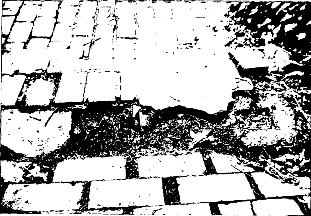
Deteriorated brick step at end of front walk
