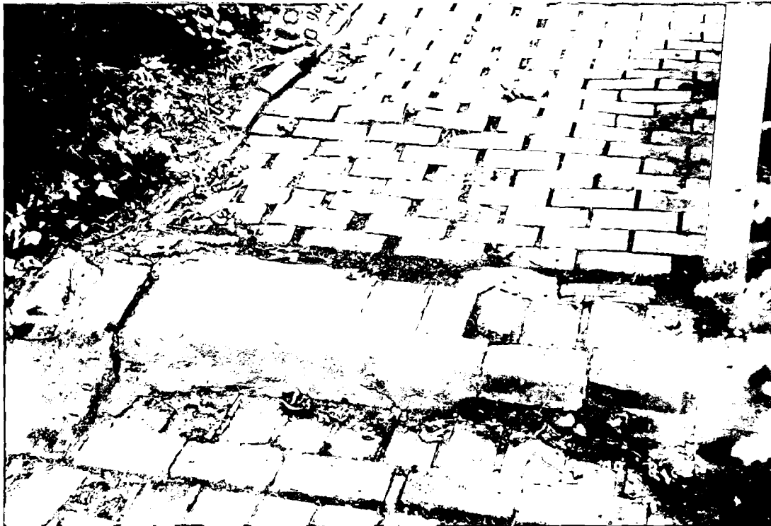
Deteriorated brick step at end of front walk
