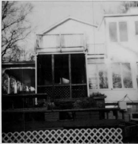
Rear screened porch SE
