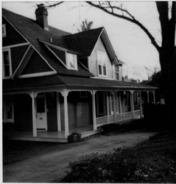
West side of house
