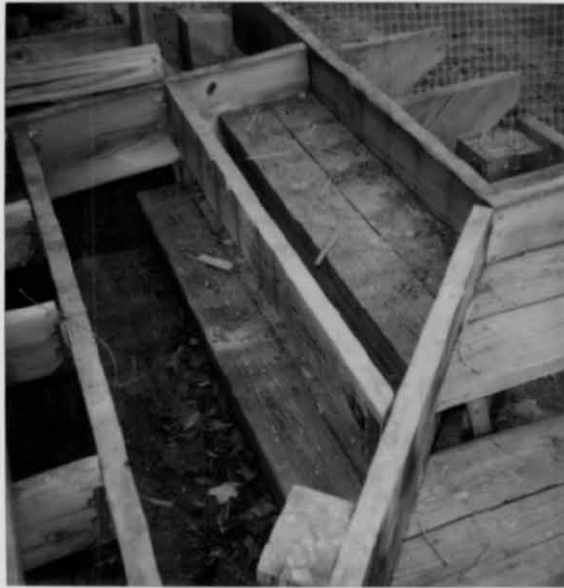
Deck, up - existing
