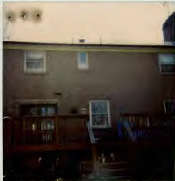
3907 WASHINGTON ST KENSINGTON - Rear Facade
