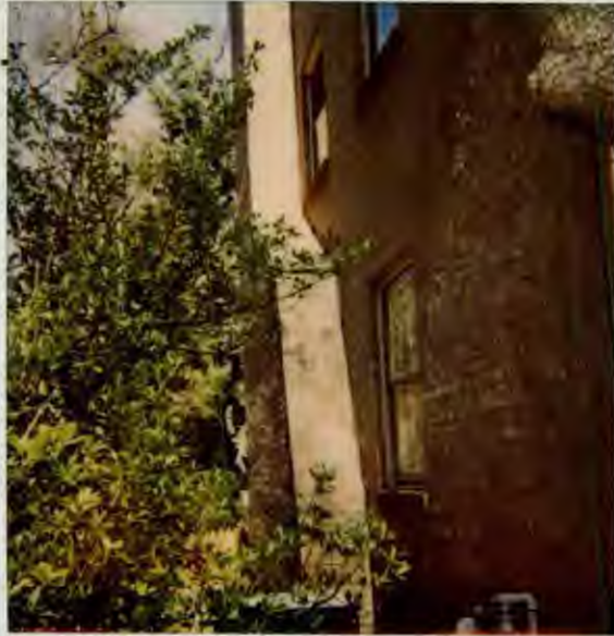
3907 WASHINGTON ST. KENSINGTON West Facade
