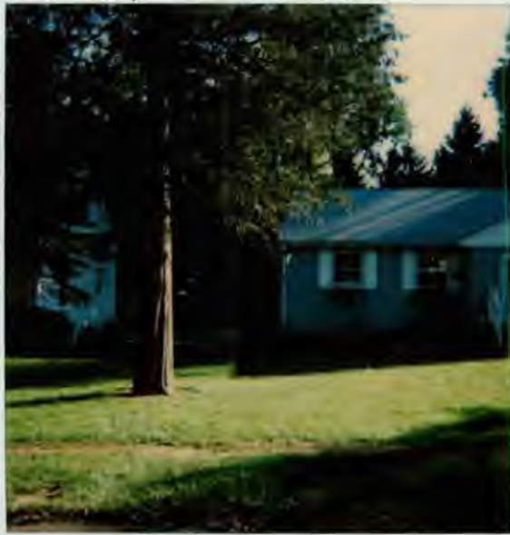
EAST SIDE OF HOUSE - FRONT VIEW
