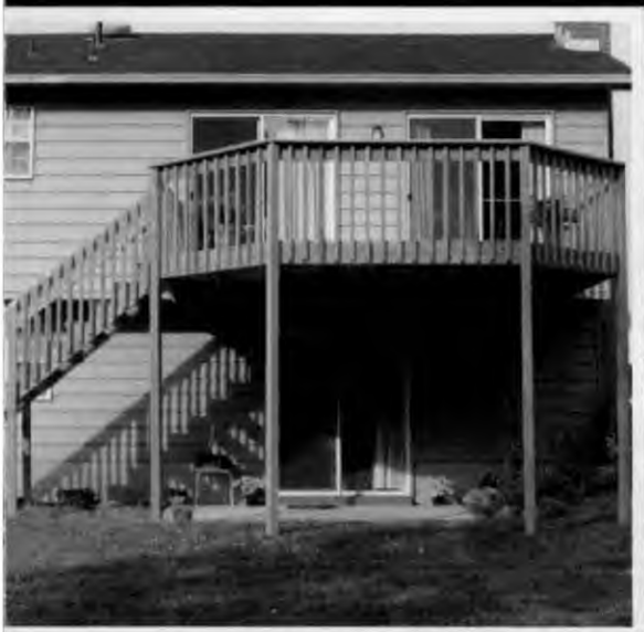
RAILING AND STEPS
