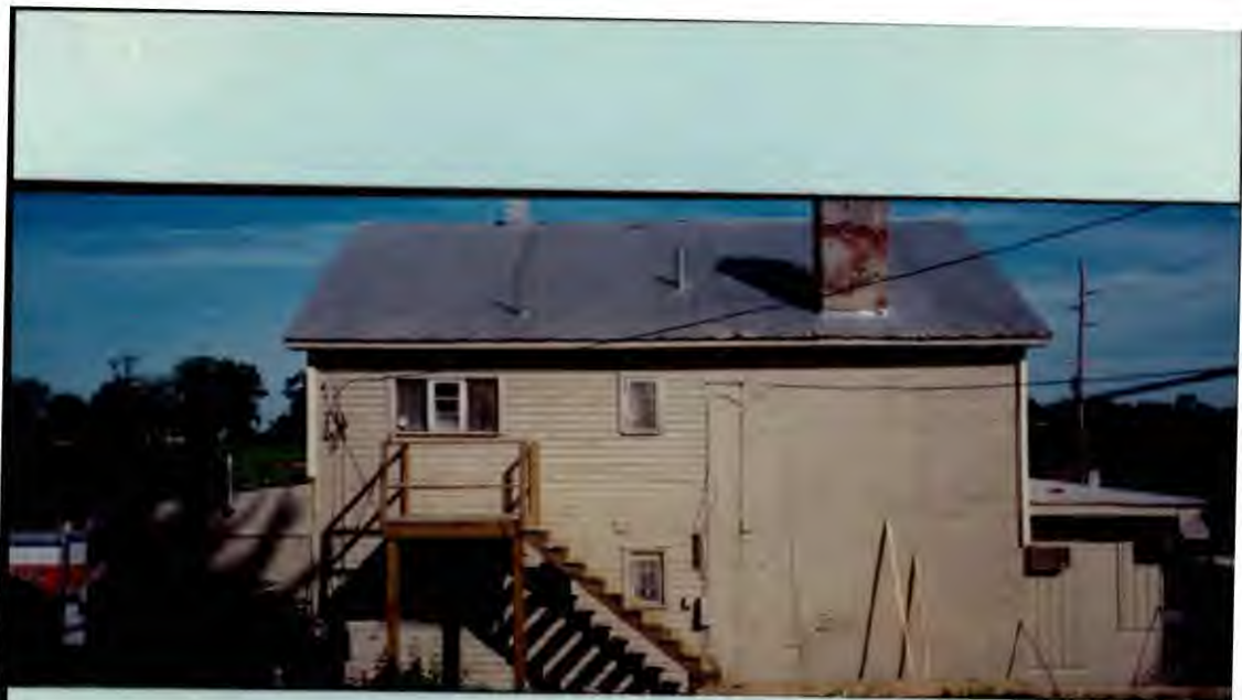
View from Ben Lewis property to North Side of Building.
