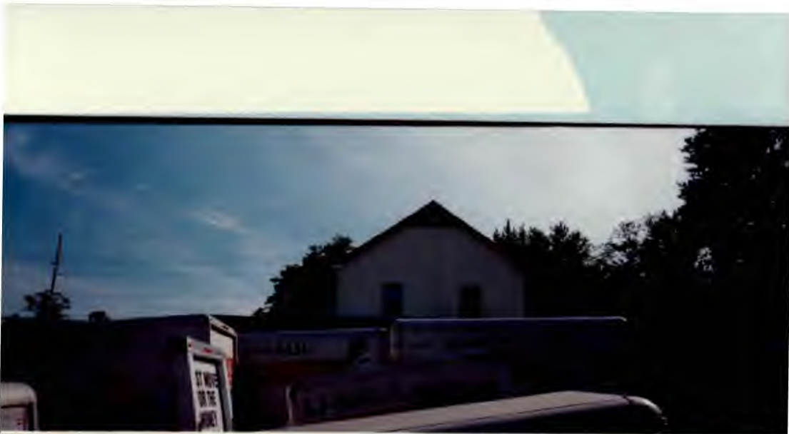
View from second Funt parcel to east side of building
