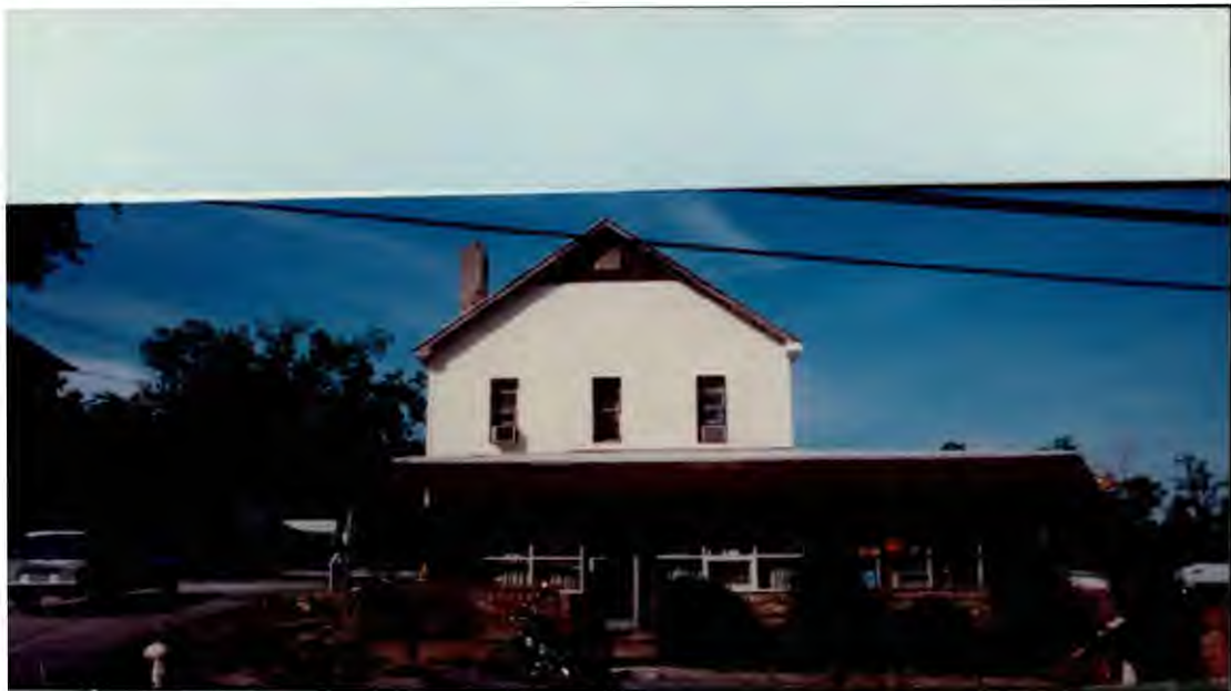
View from across St 355 ( Citizens Bank Property ) to West side of building, and Duane lot
