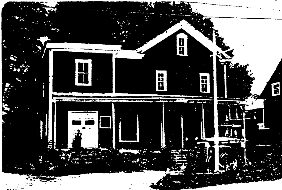
Willson Store, 13/10 Facade: West Taken by: Kevin Parker. 1979
