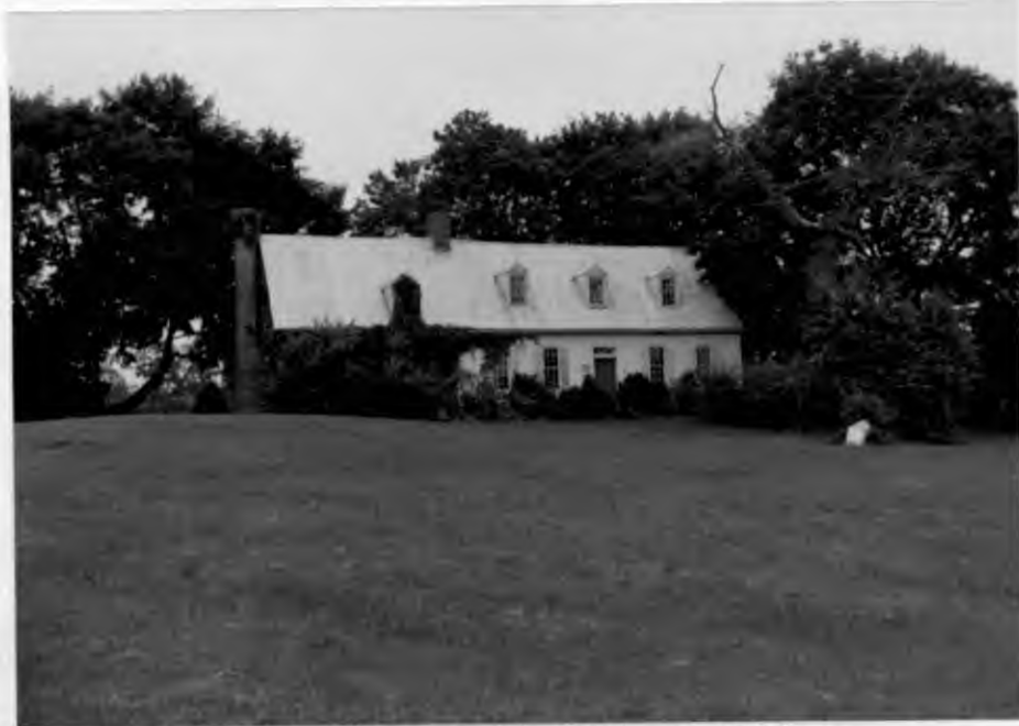
Front View of Historic Dwelling
