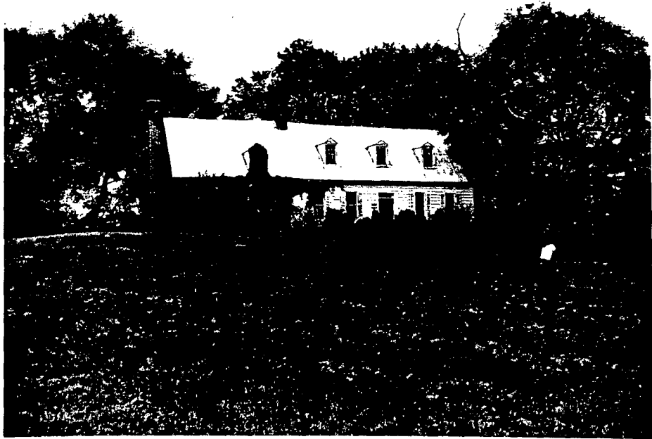
Front View of Historic Dwelling
