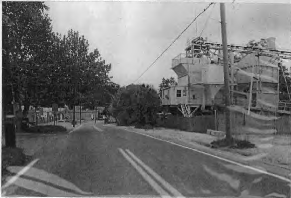
14 MERIT CONCRETE - METROPOLITAN AND WHEATLEY
