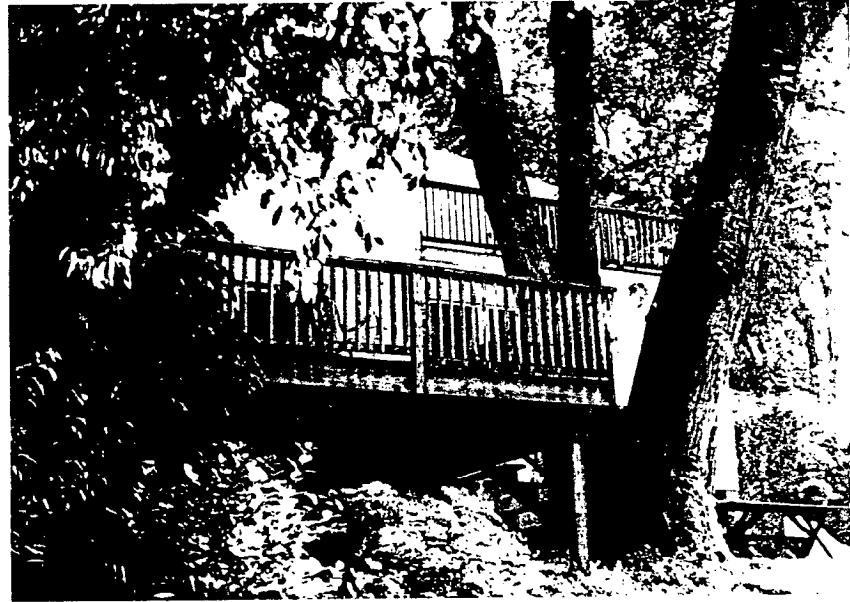
ADJOINING NEIGHBOR'S DECK
