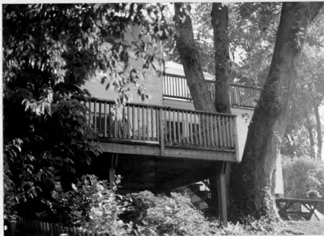
ADJOINING NEIGHBOR'S DECK
