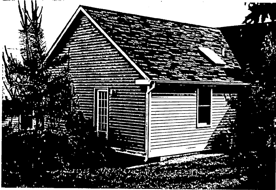
① BLDG. CORNER & PROPOSED ADDITION
