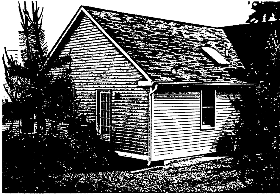
① BLDG. CORNER & PROPOSED ADDITION
