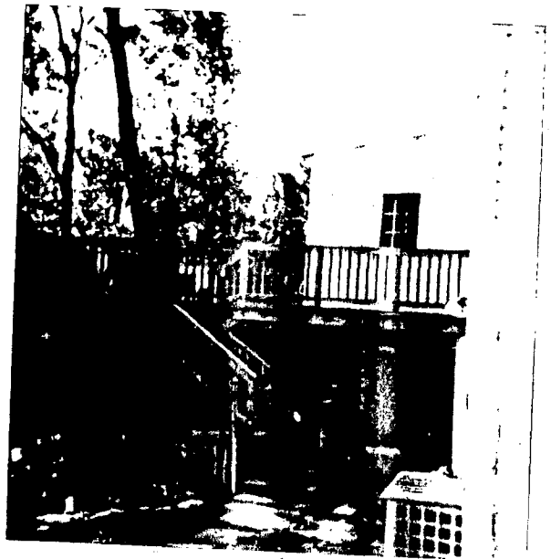
North side in back yard
