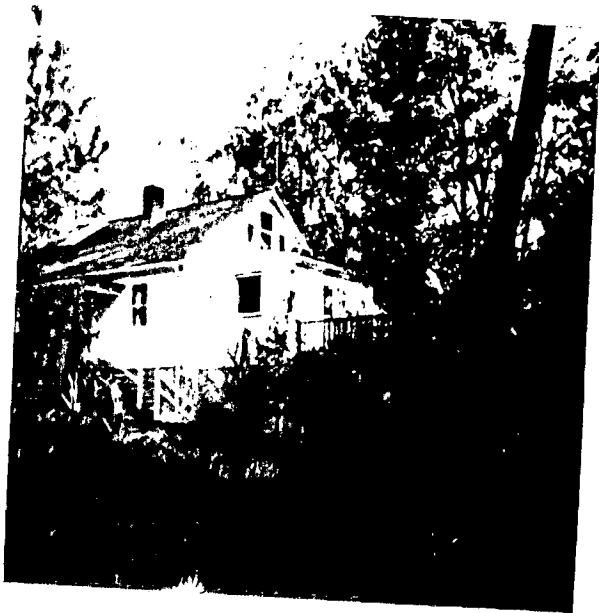
South side From back yard
