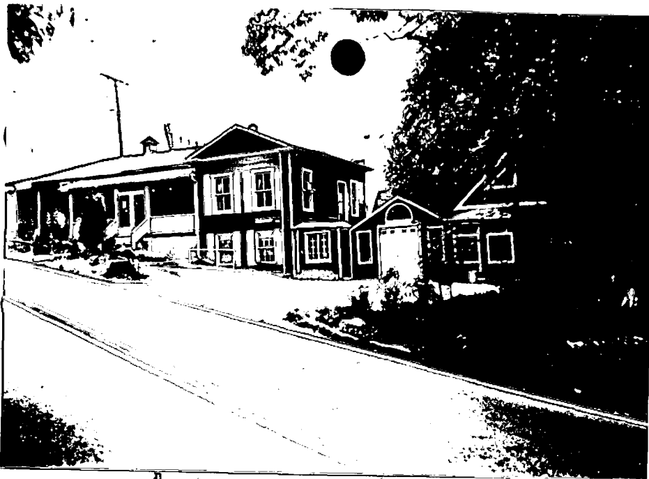
VIEW FROM CAPITOL VIEW AVE. LOOKING SE SHOWING EXISTING AND LOCATION OF PROPOSED PORCHES
