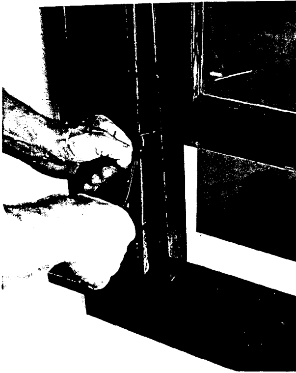
1 Gently remove the sash stops using a pry bar or putty knife. In some cases they are screwed on. Save them as they will be reinstalled when the job is completed.
