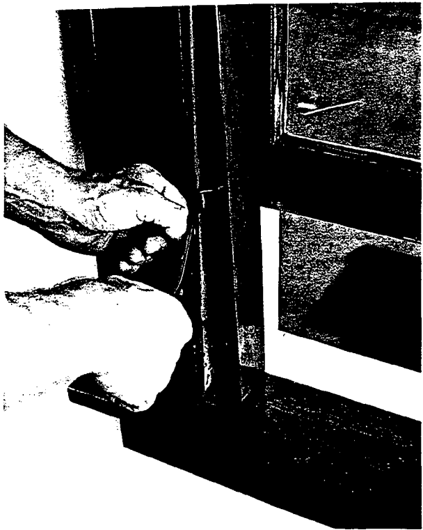
1 Gently remove the sash stops using a pry bar or putty knife. In some cases they are screwed on. Save them as they will be reinstalled when the job is completed.
