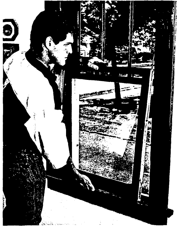
2 Now lift the bottom sash out. If your windows are rope and pulley operation, cut the rope and remove the pulley and counter weights.
