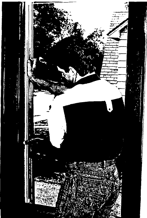
7 Snap the jambliners in place over the jambliner clips.
