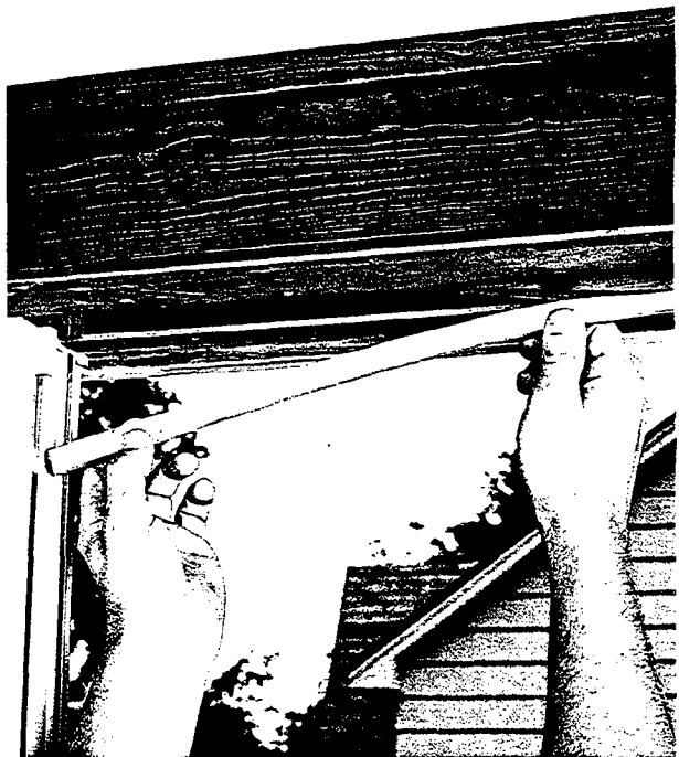
8 Press the vinyl head parting stop into the same channel that the old parting stop came out of. NOTE: Make sure the flexible fin is to the outside.
