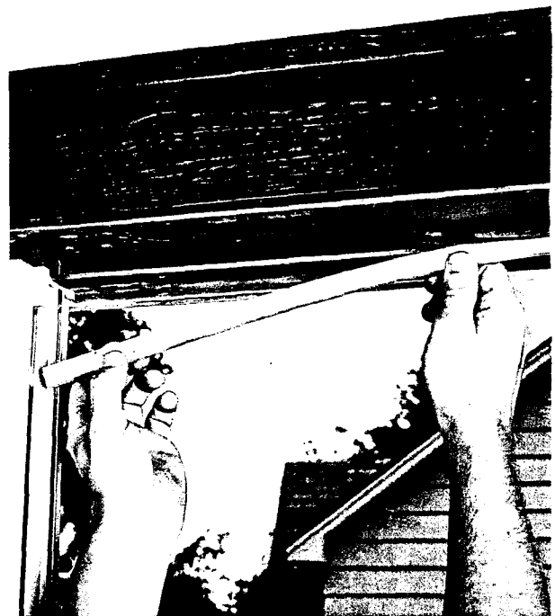
8 Press the vinyl head parting stop into the same channel that the old parting stop came out of. NOTE: Make sure the flexible fin is to the outside.
