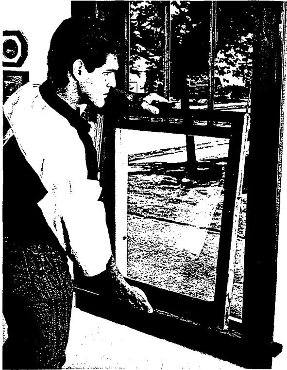
2 Now lift the bottom sash out. If your windows are rope and pulley operation, cut the rope and remove the pulley and counter weights.
