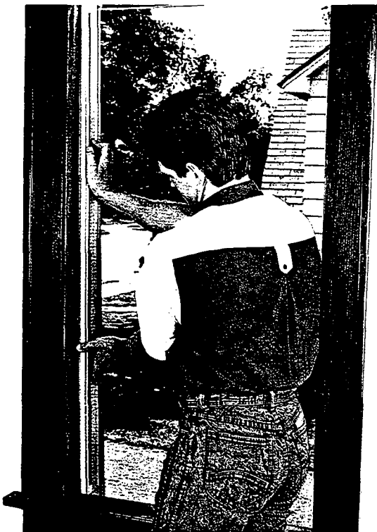
7 Snap the jambliners in place over the jambliner clips.
