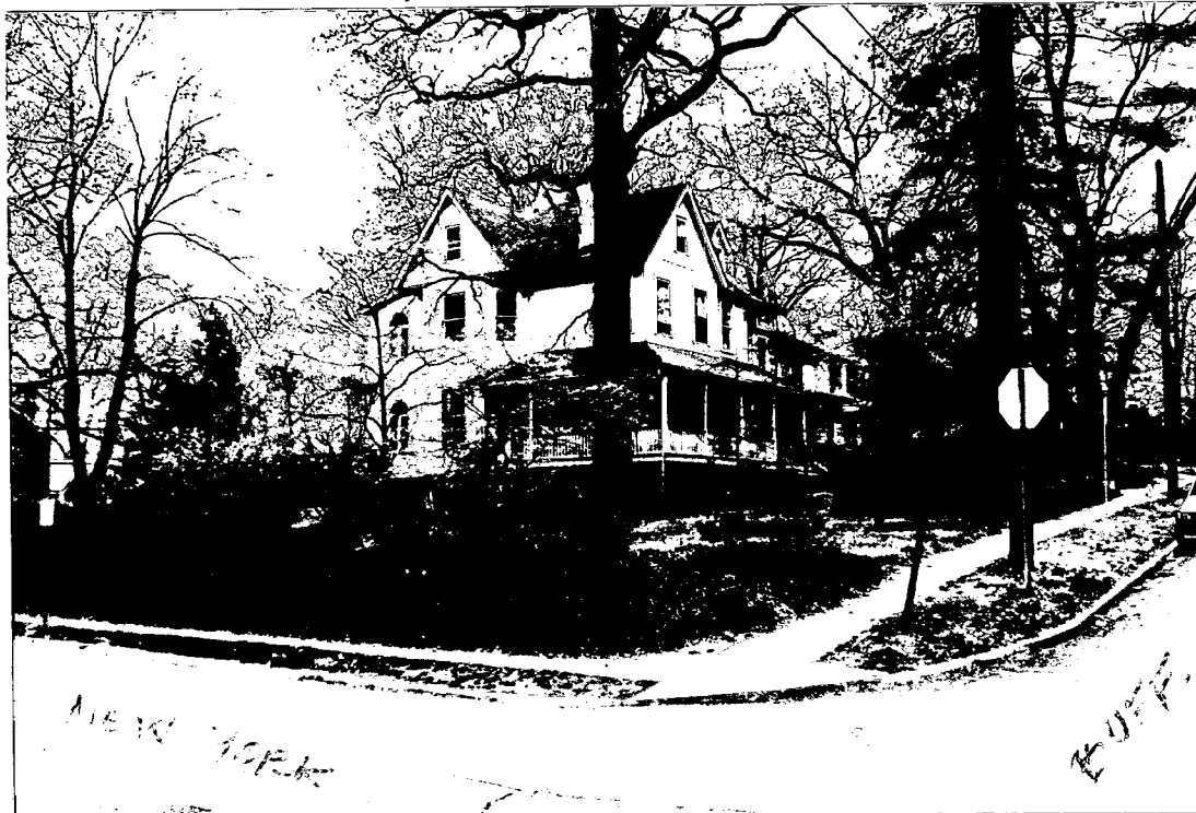
OPPOSITE E LEFT OF 511 NY AVE
