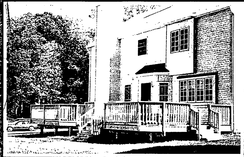
DECK—with railing and steps
