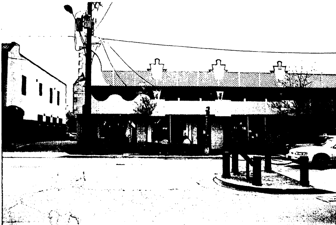
Laurel Avenue - Existing Facade
