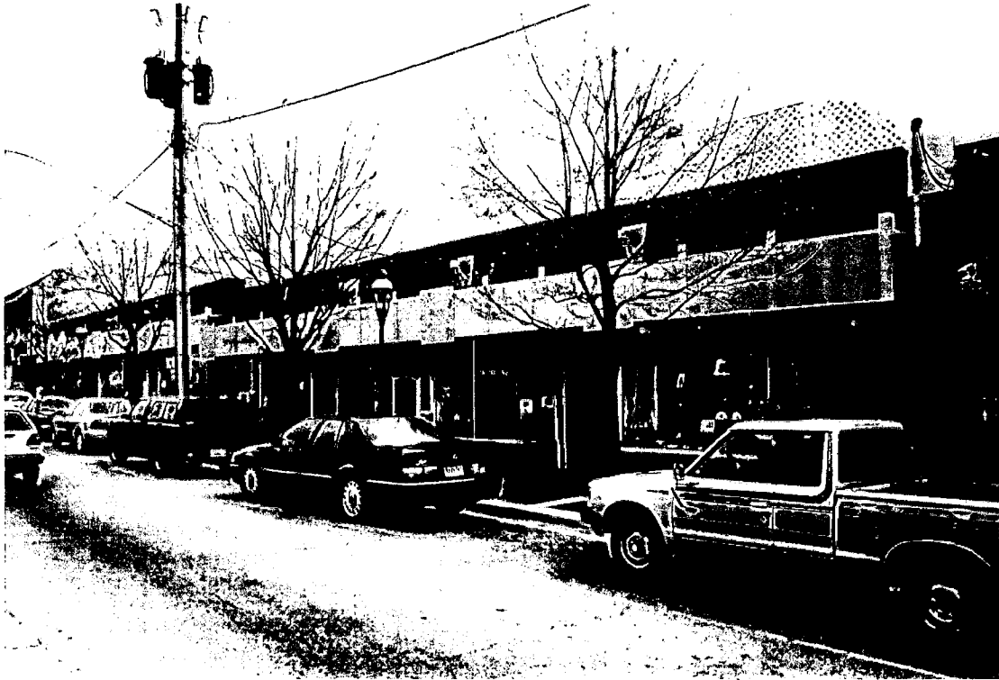
Laurel Avenue - Existing Facade
