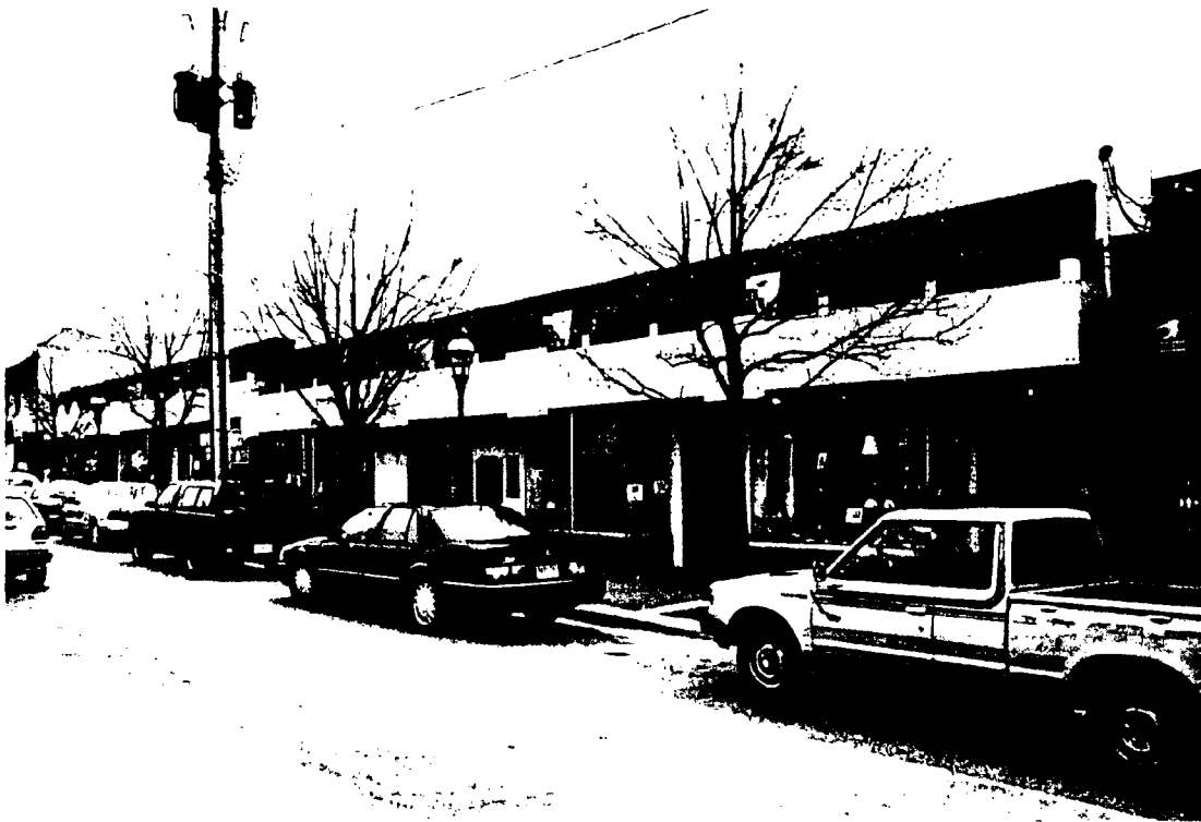
Laurel Avenue - Existing Facade
