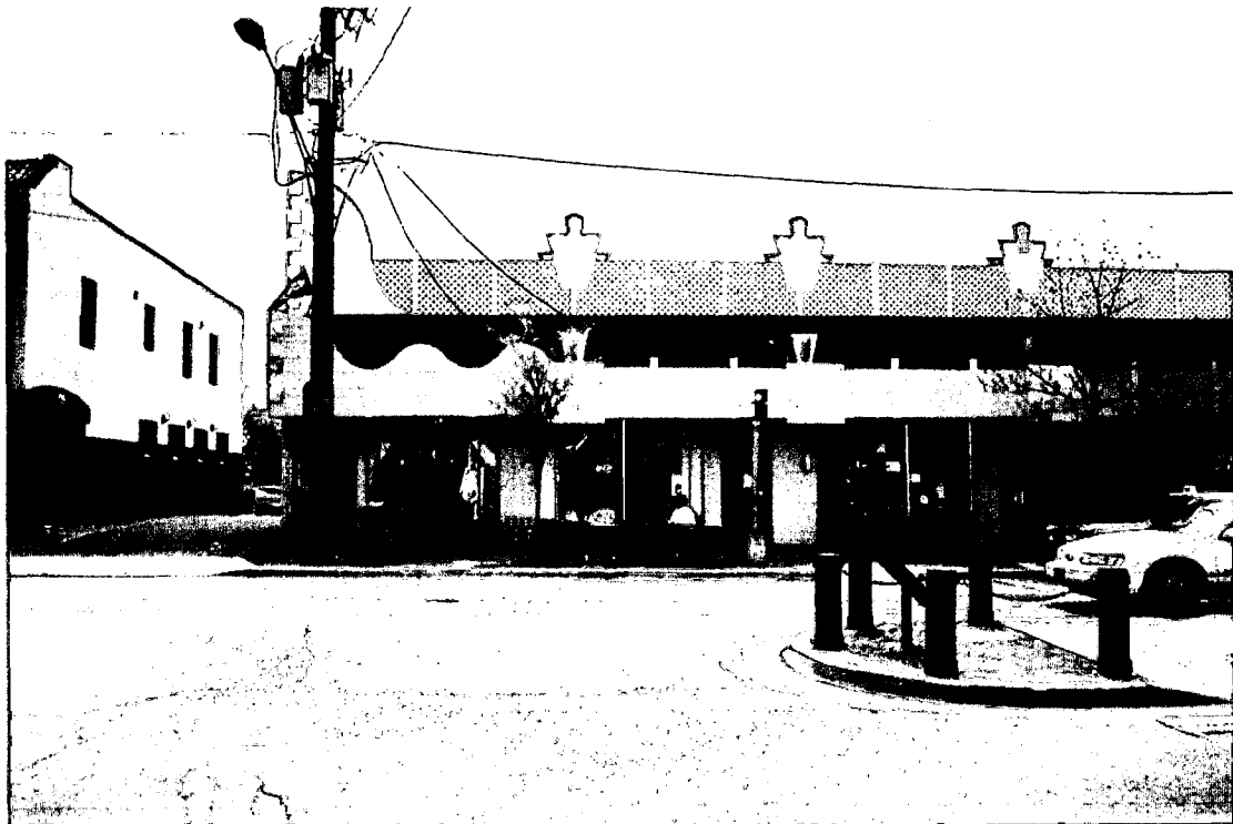
Laurel Avenue - Existing Facade
