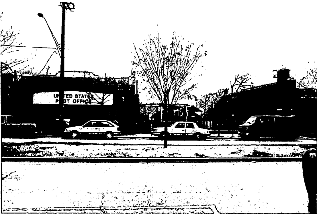
Laurel Avenue - Existing Facade
