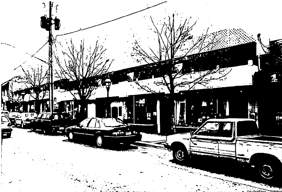
Laurel Avenue - Existing Facade
