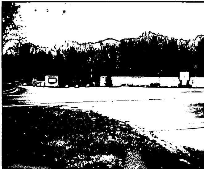
View of entrance looking North
