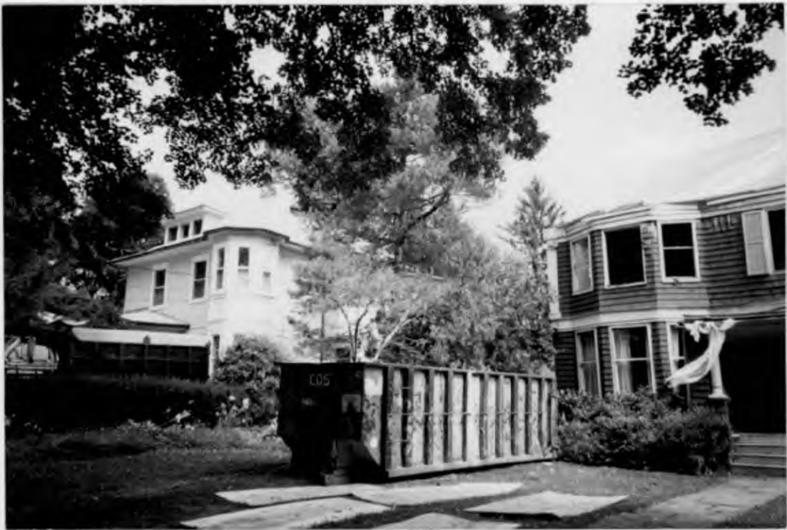
SOUTH-EAST CORNER OF HOUSE AS VIEWED FROM NEIGHBORING PROPERTY
