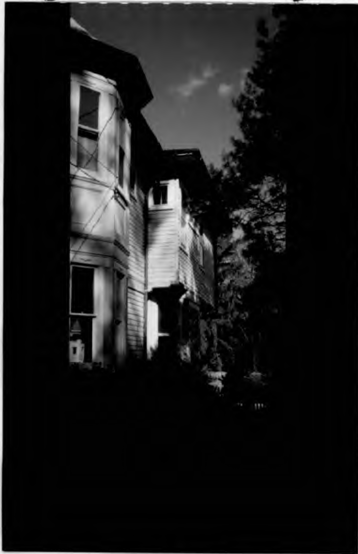
EAST SIDE OF HOUSE, LOOKING NORTH NORTH-WEST
