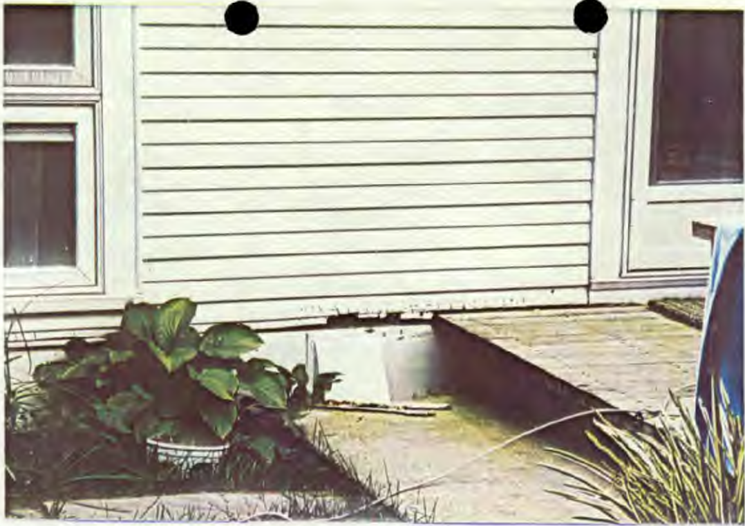
Typical water damage at North Elevation
