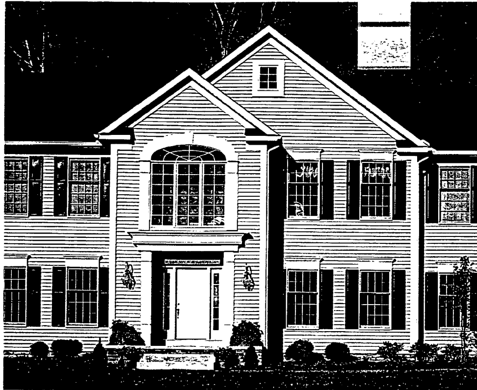
Profile: Clapboard Exposure: Double 4" Butt edge: 1/2"
