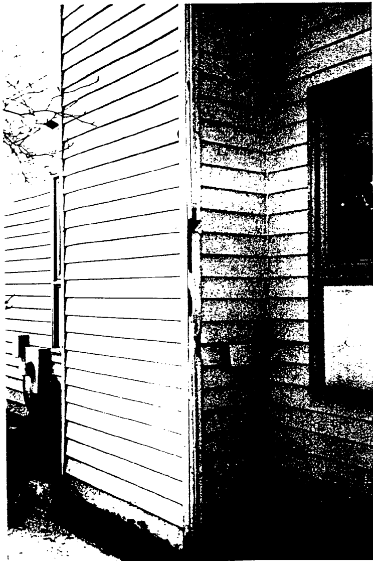
DETAIL OF RHS CHIMNEY AND REPRESENTATIVE DAMAGE
