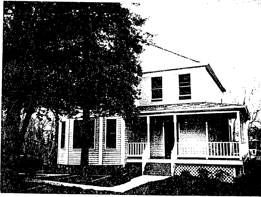
Photos of Porch As Built
