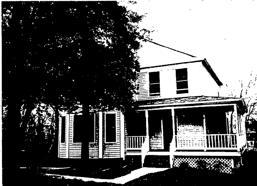
Photos of Porden As Built
