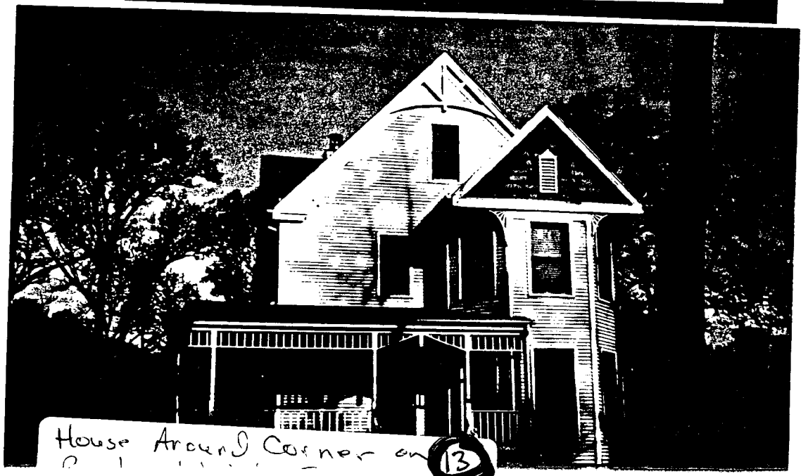
View of 2 Story Houses on Grant & Barker - View from 10003 Grant
