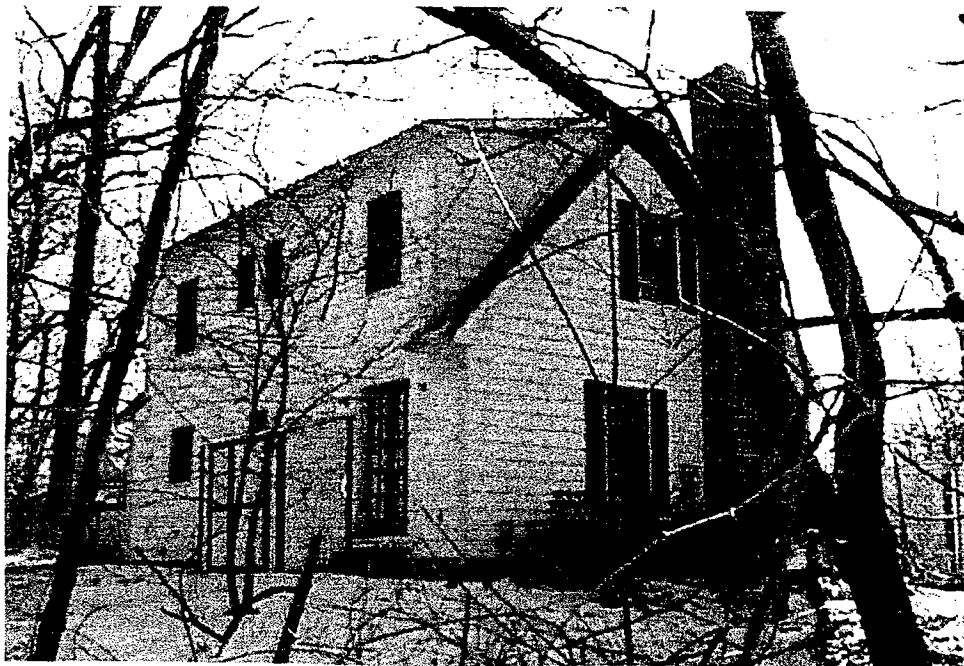
CORNER VIEW: NORTH
