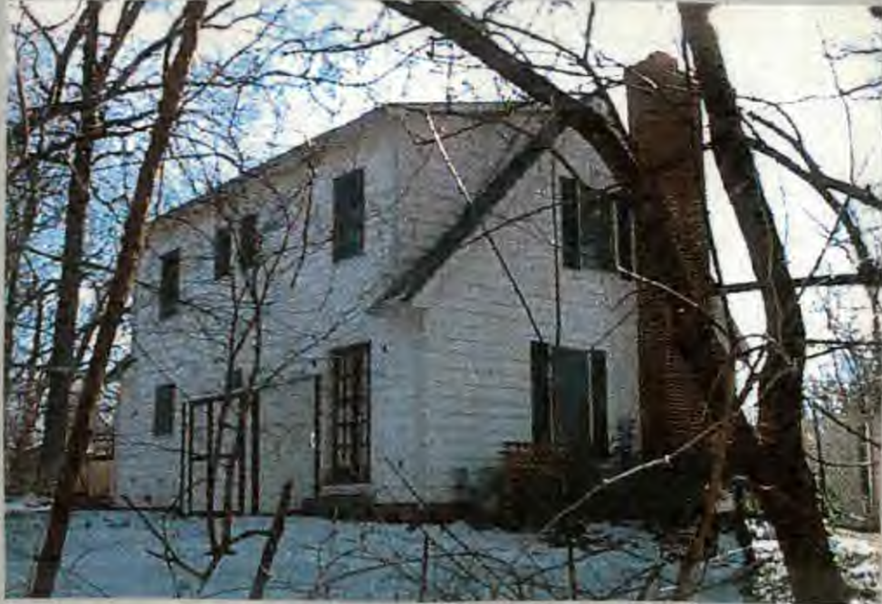
CORNER VIEW: NORTH
