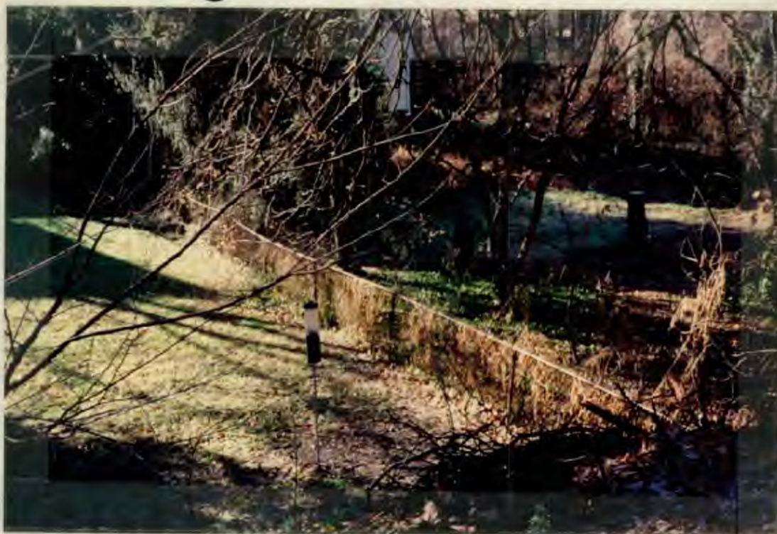
Existing chain link fence which is approximately four feet inside the property line.
