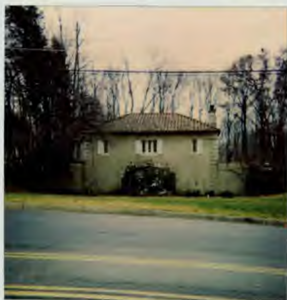
Marwood Gatehouse North Side (facing River Rd.)
