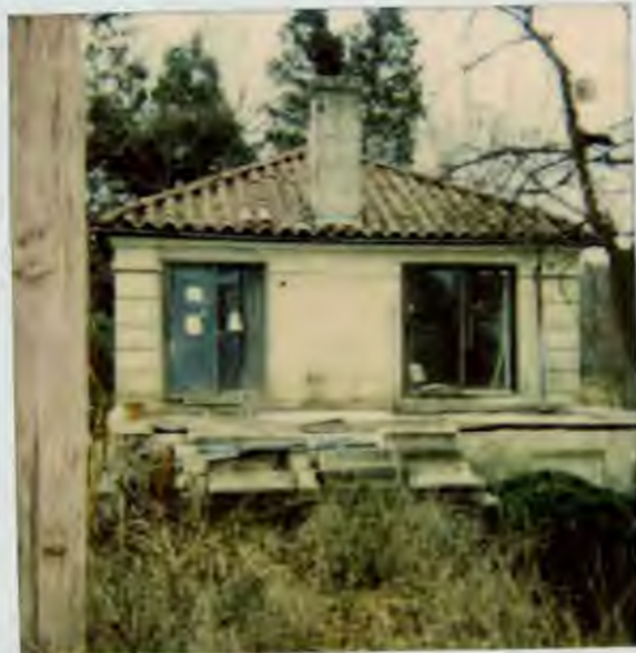
Marwood Gatehouse West side facade
