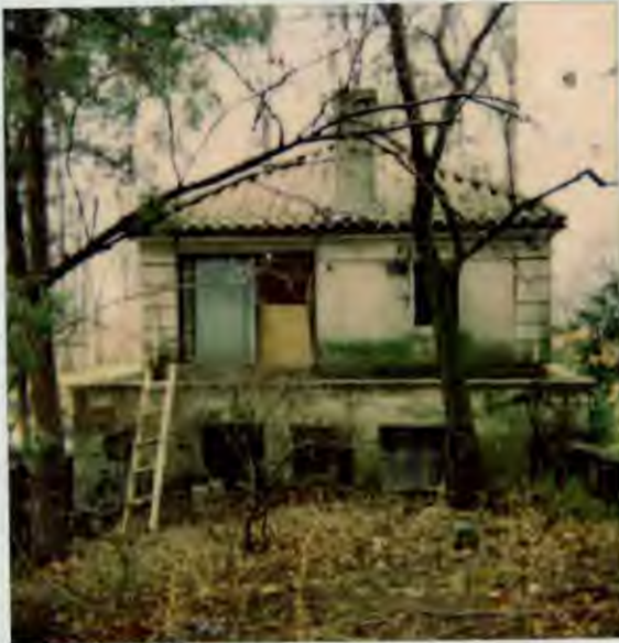
Marwood Gatehouse East side
