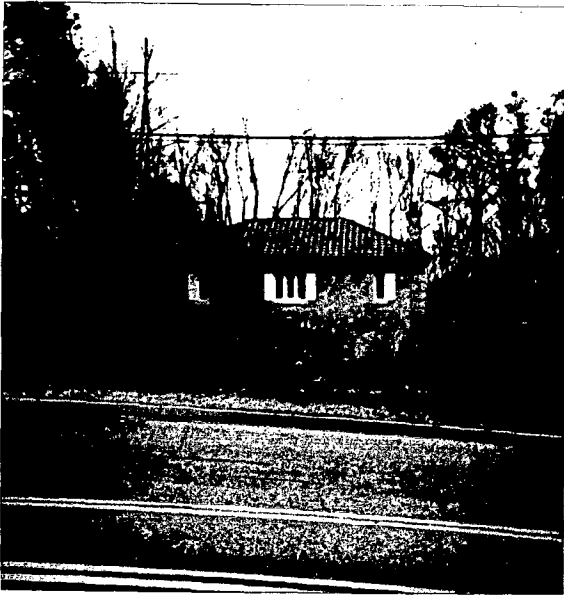
Marwood Gatehouse North Side (facing River Rd.)
