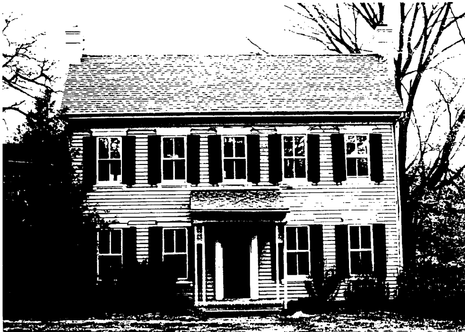
EXISTING NORTH ELEVATION BUILDING FACE TO RIGHT OF WAY
