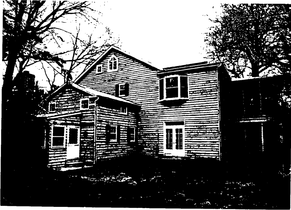
BUILDING FACE TO SOUTH PROP.
