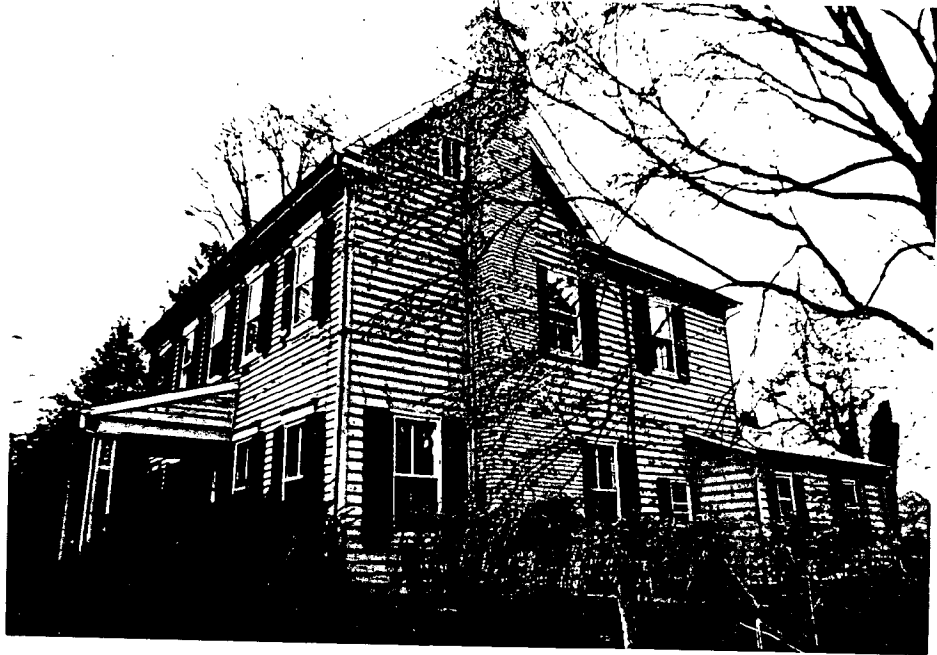
BUILDING FACE TO WEST PROPERTY
