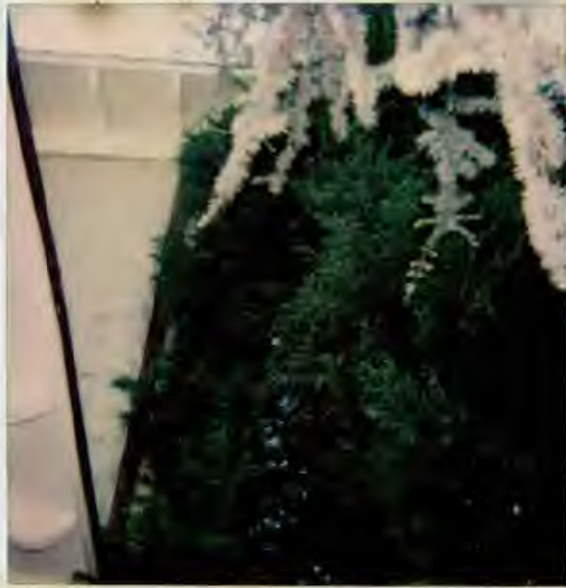
Tree growing in to building
