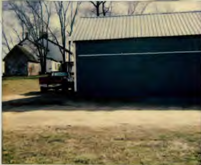
BLDG. SITE SOUTH VIEW
