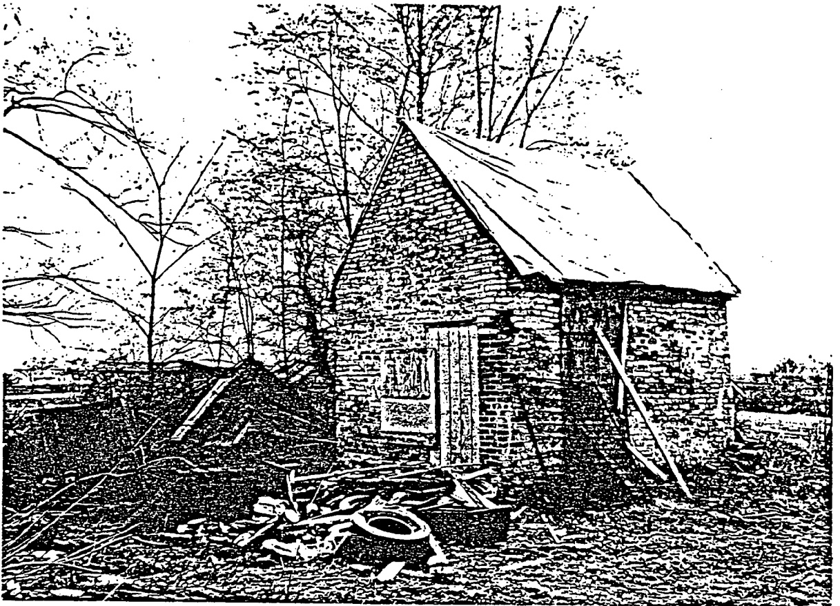
Smokehouse of pierced brick con- struction. South & East facades.
