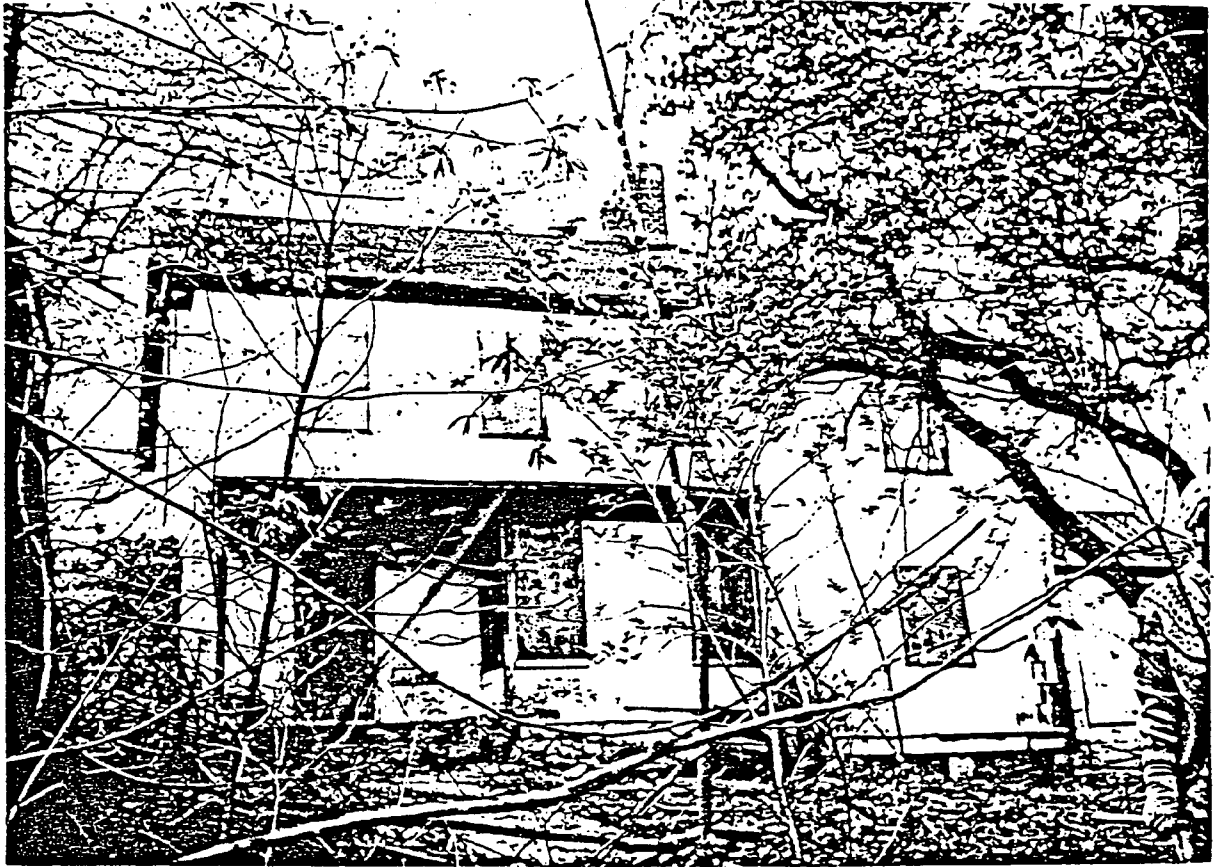
East facade of 3 bay main block and 1855 addition
