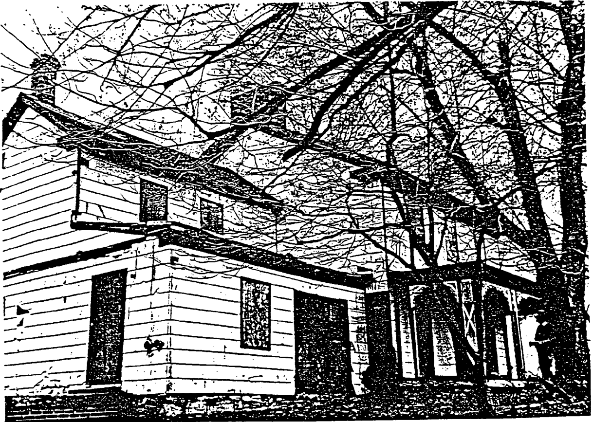
North & West facades of house. Main block 1826-40, 1 1/2 story North wing. 1855 addition Double chimney, north side of main block, serves 5 fireplaces.
