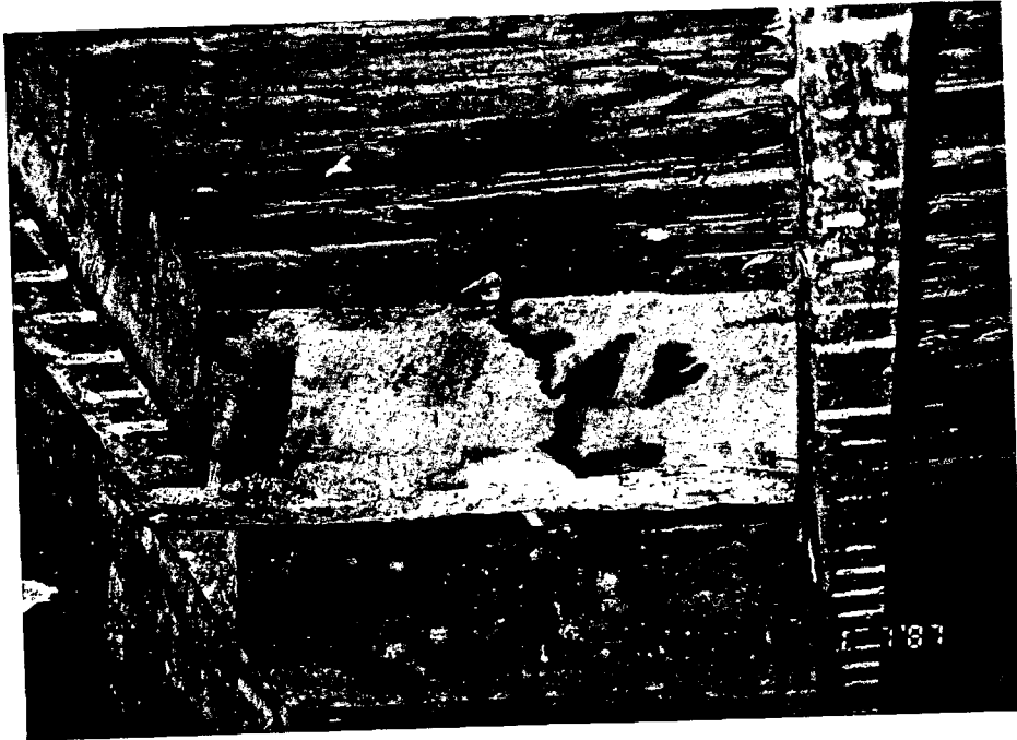
Braces holding south chimney Braces holding south chimney
