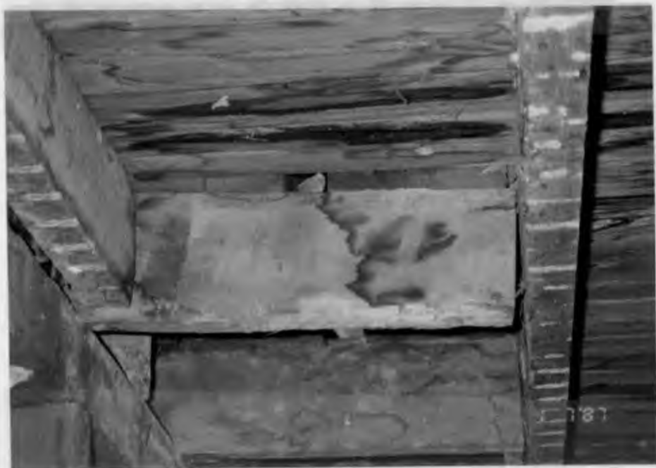
Braces Holding South Chimney
