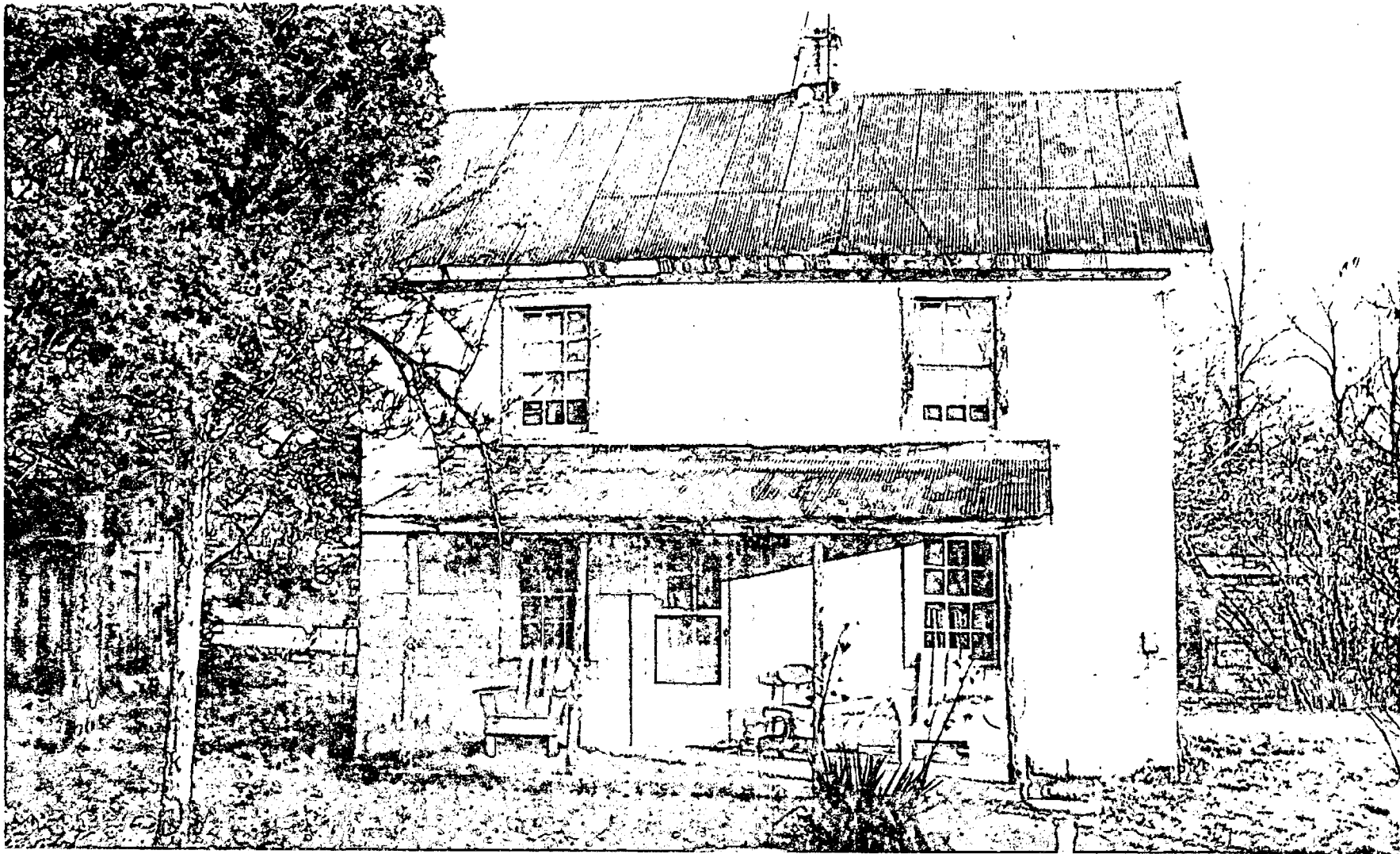
Figure 42. Duffin Hebron House, White Grounds. This two story frame house was constructed, according to family tradition, by Henry Duffin, a former slave, in the 1870's on land that he purchased. Its basic two room down and two room up floor plan is similar to that of most houses of black landowners of the 19th century, whether of log or frame construction.
