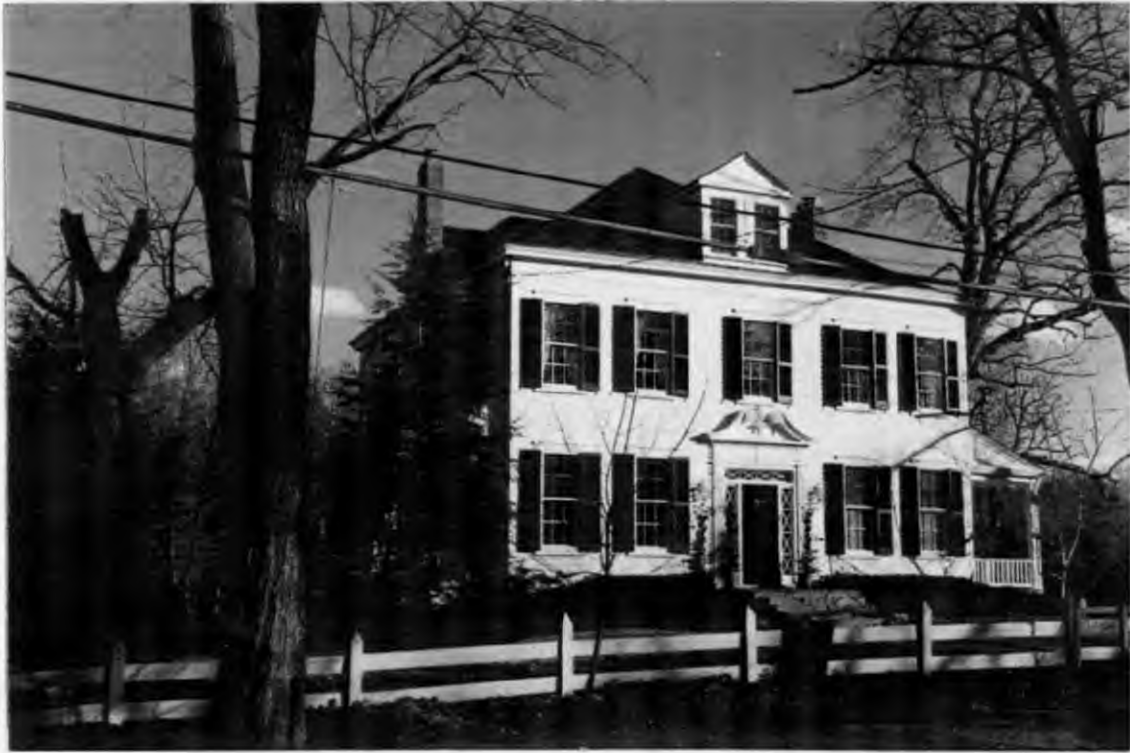
1. Northwest Corner - Front Elevation - Montgomery Avenue :
