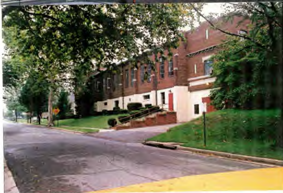
6. Armory Avenue (West side)
