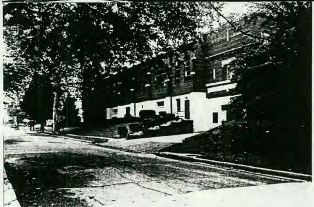
6. Armory Avenue (West side)
