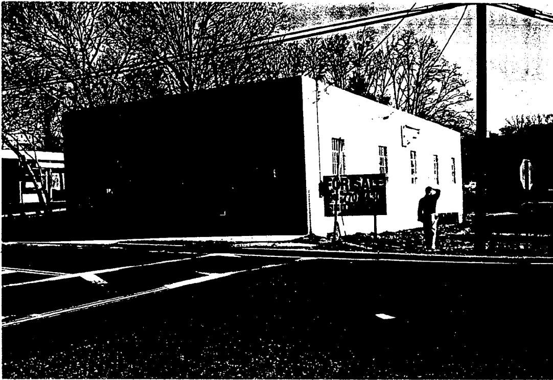
SOUTHEAST CORNER ELEVATION
