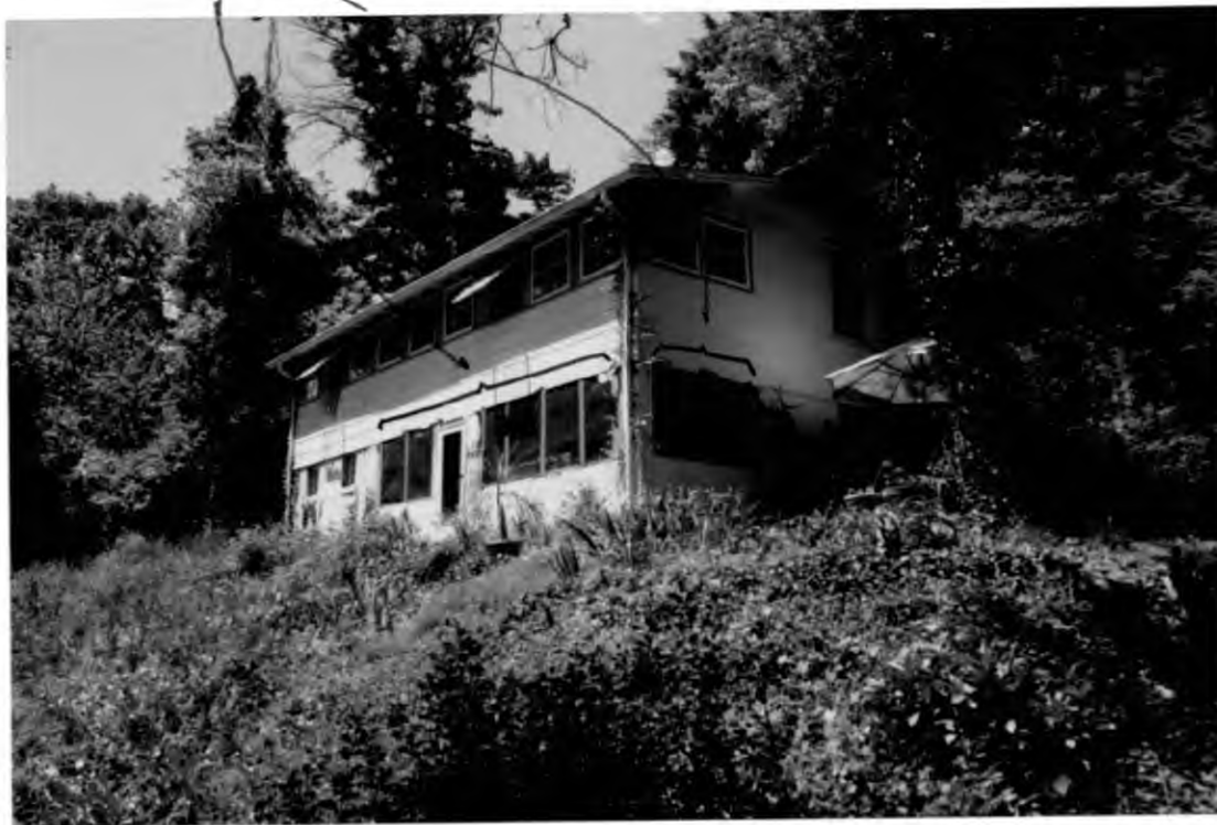
Side view - South and East Elevation
