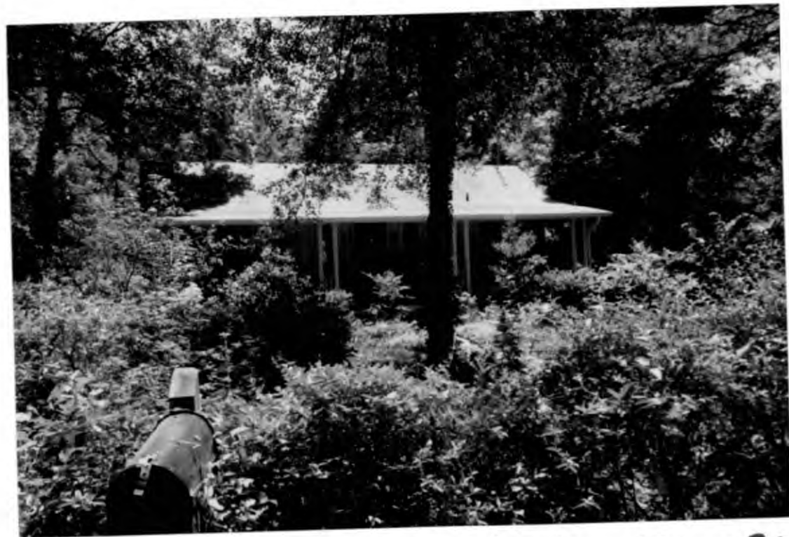
Front View - North Elevation
