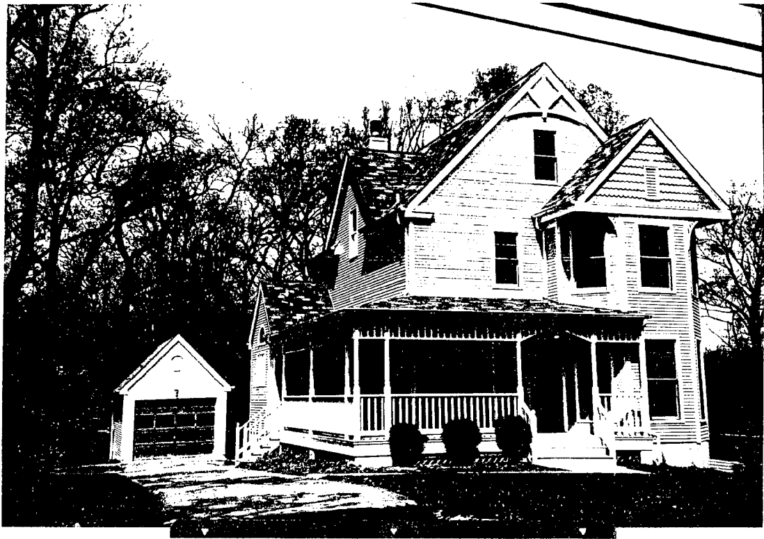
South Side of House
