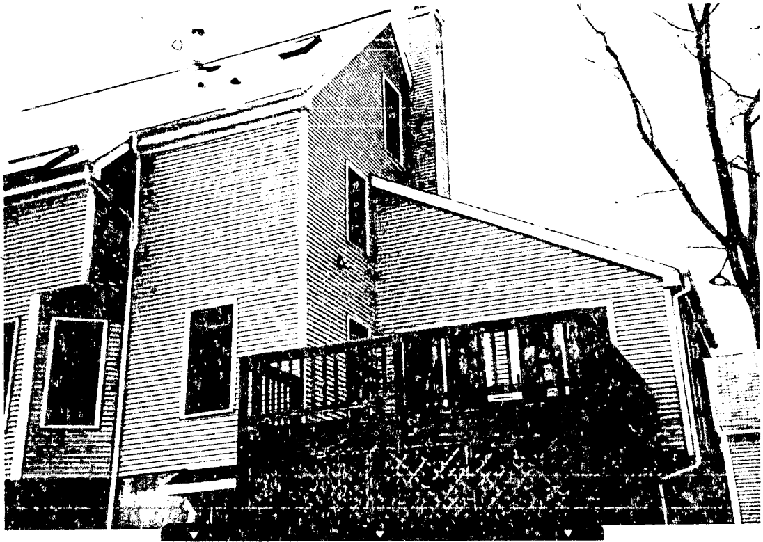
Detail: Porch Area
