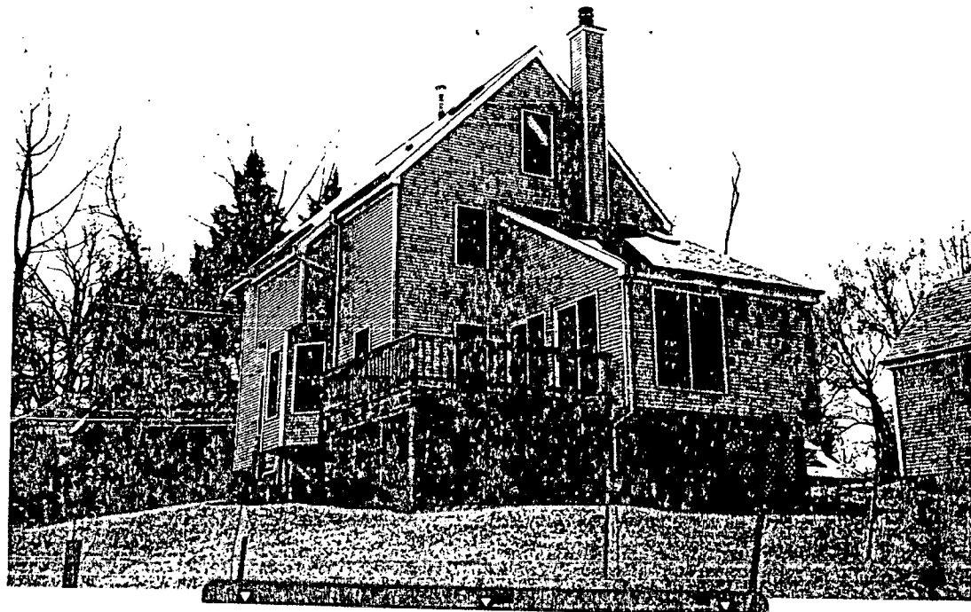
North/East Sides of House (from adjoining property)
