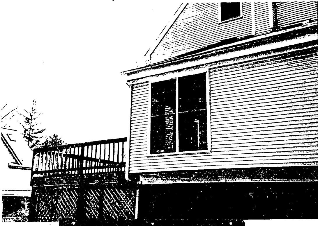
North Side of House (Detail of Deck Area)
