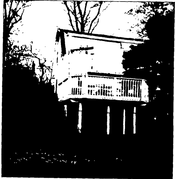
View of S.E. side of 2911 Barker (View from proposed shed to house)
