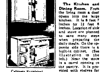
Cabinets Furnished in Kitchen
