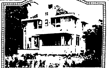
Alhambra The millwork and other materials furnished are certainly of very exceptional quality. 5925 Nina Ave., Norwood Park, Ill.
