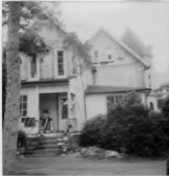
4710 Waverly Ave. rear elevation from own private yard
