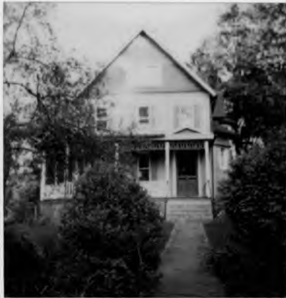
4710 Waverly Ave. front elevation from public right of way
