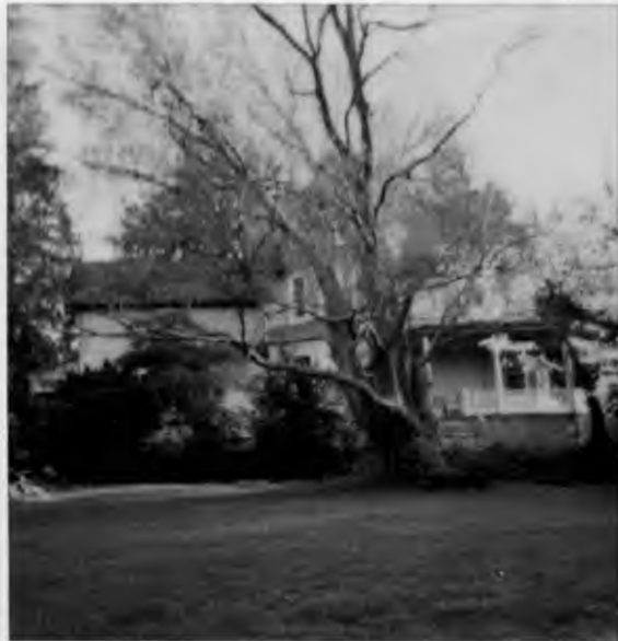
4710 Waverly Ave. right elevation from own private yard
